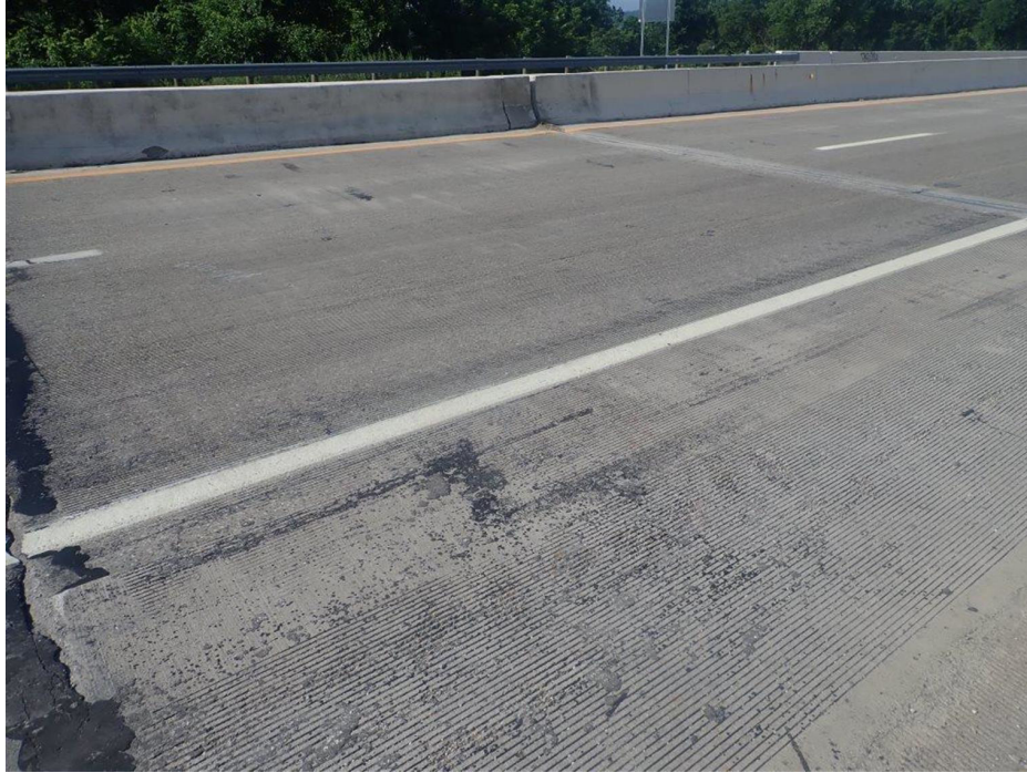
PHOTO 8 Condition Description Forward approach slab, southbound lanes shown (looking southeast)
