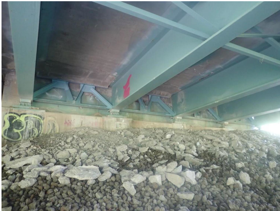
PHOTO 1 Description Rear Abutment, north elevation, southbound lanes (looking south)
