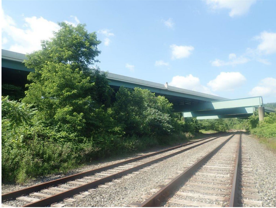
PHOTO 2 Elevation, Condition Description West elevation (looking southeast)
