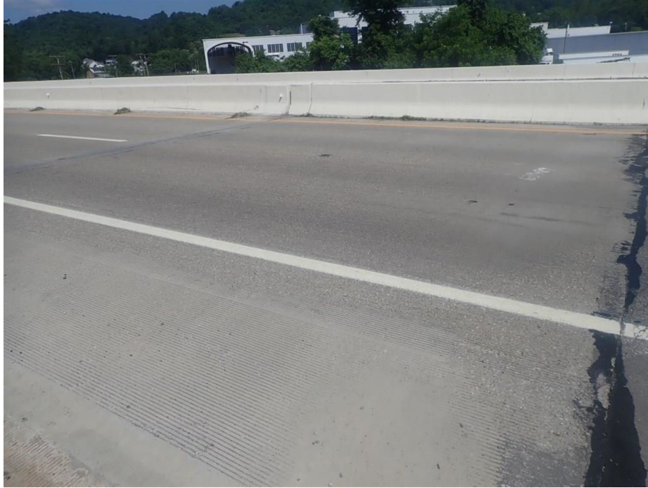
PHOTO 19 Condition Description Forward approach slab, northbound lanes shown (looking southwest)
