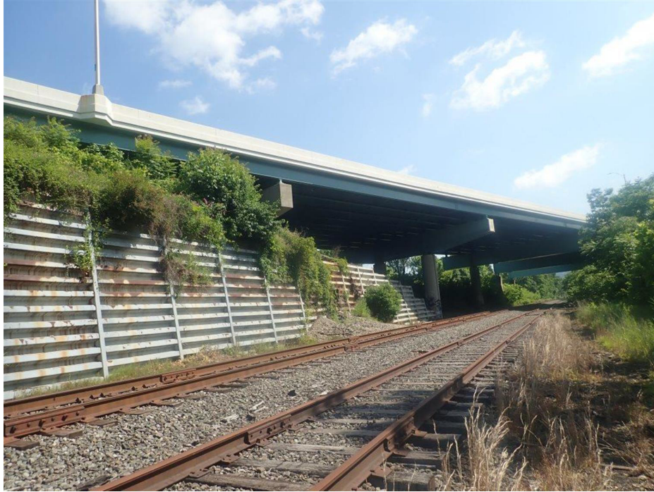
PHOTO 1 Elevation, Condition Description East elevation (looking northwest)
