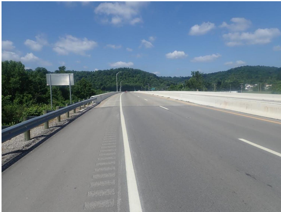
PHOTO 3 Description Forward end view, northbound lanes (looking south)
