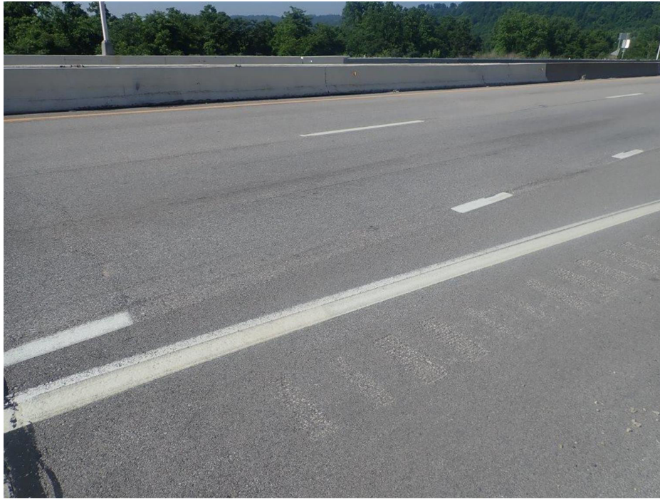
PHOTO 3 Condition Description Rear approach wearing surface, southbound lanes shown (looking southeast)
