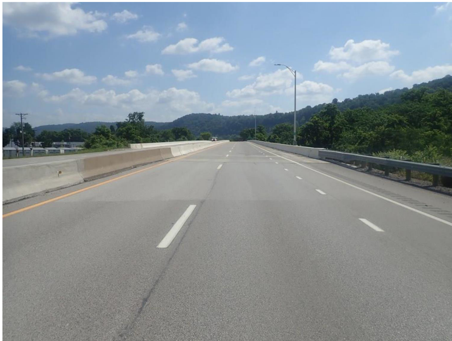
PHOTO 1 Description Rear end view, northbound lanes (looking north)
