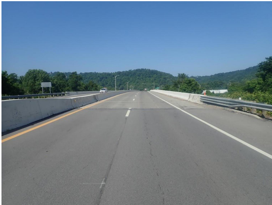
PHOTO 2 Description Forward end view, southbound lanes (looking south)
