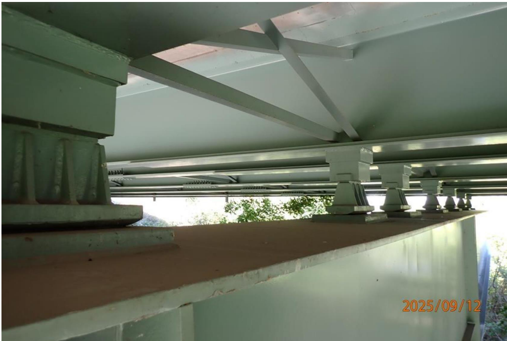
PHOTO 8 Description West rocker bearings at Pier 2 (looking southwest)
