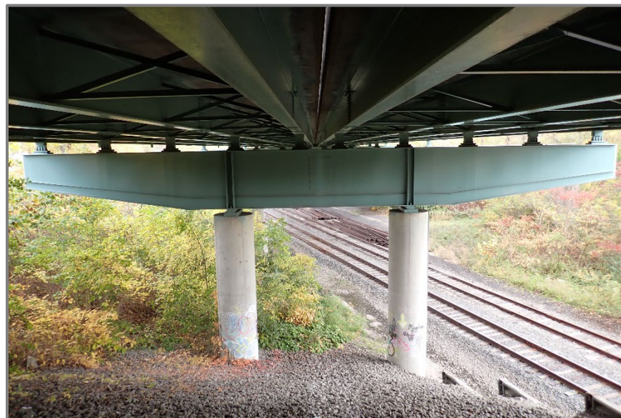
Figure 4 – Pier 1 cap south elevation (typical hammerhead-style pier), looking north.
