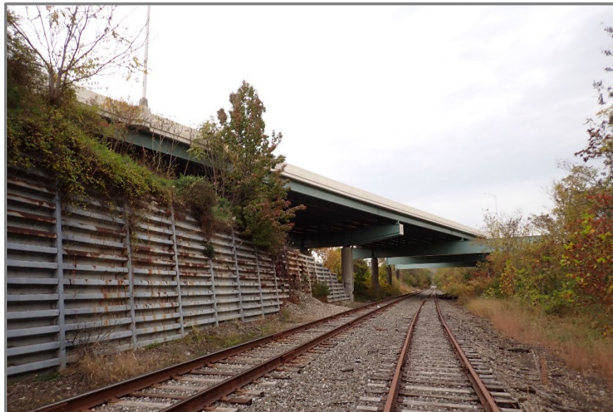
Figure 1 – BEL-7-1187 east elevation, looking northwest.
