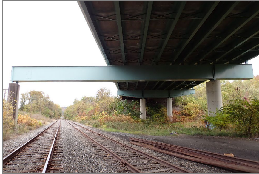
Figure 5 – Pier 4 cap south elevation (typical straddle pier), looking north.
