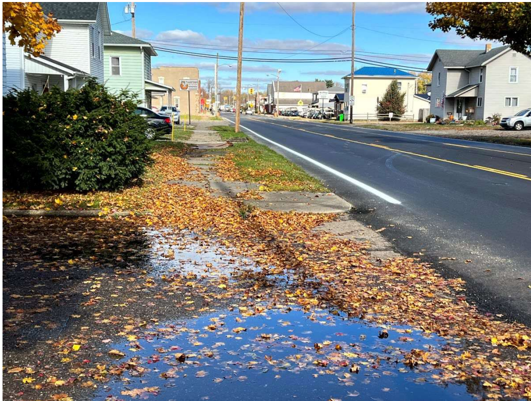
Photo 2: Intersection of Wooster Avenue and 2 nd St SW.
