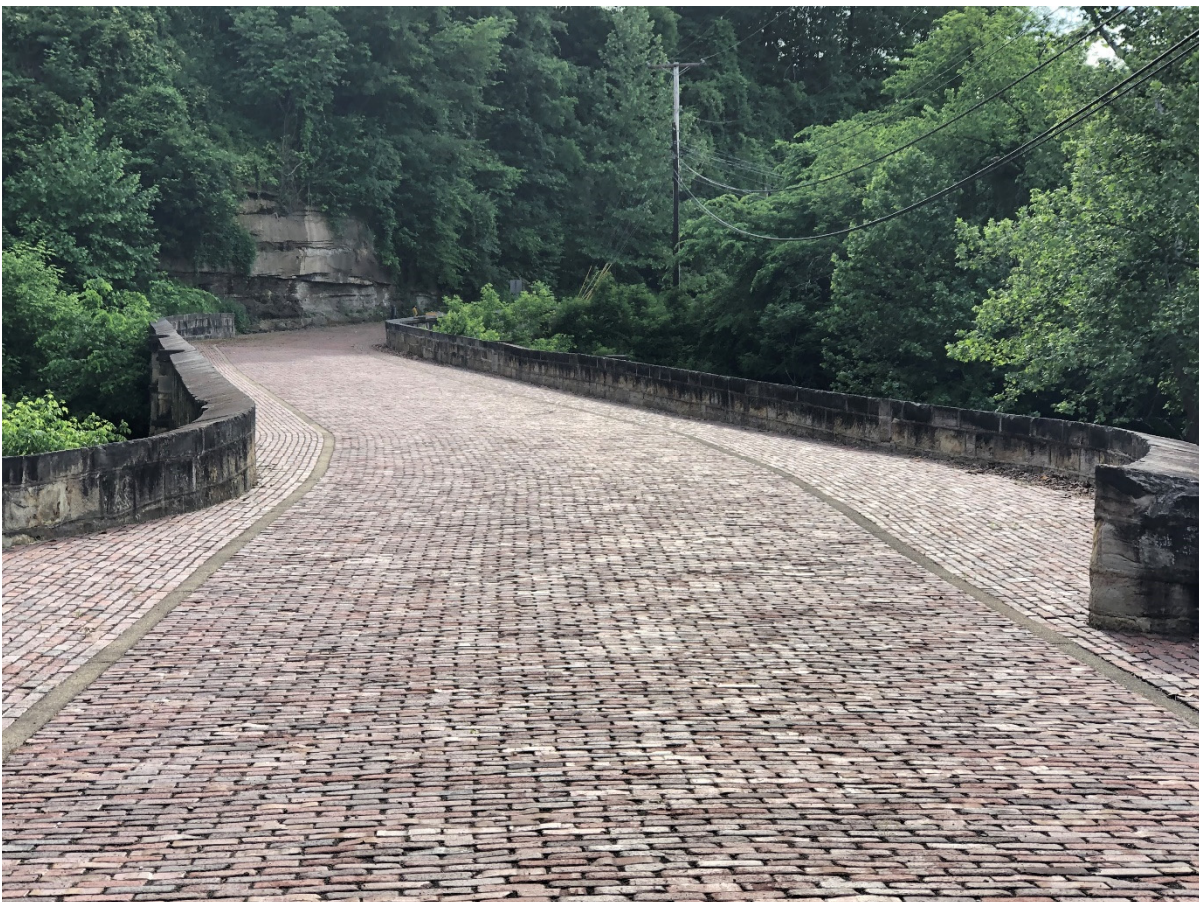
Historic Blaine “S” Bridge
