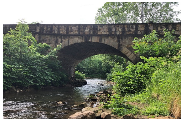
Wheeling Creek under the Historic Blaine "S" Hill Bridge
