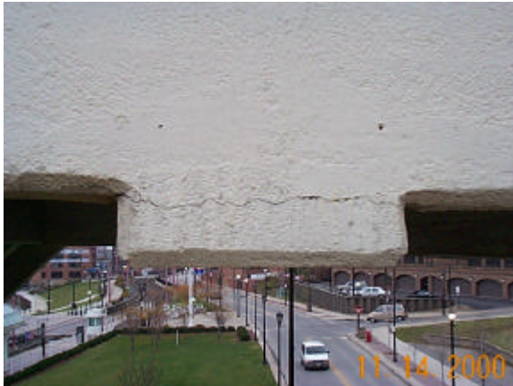
Photo 28 – Span 12, Floorbeam 5, South Face dcp00248jpg
