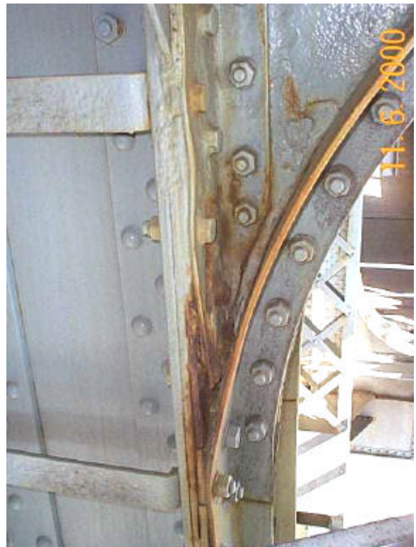
Photo 52 - South Arch at panel point 1'
