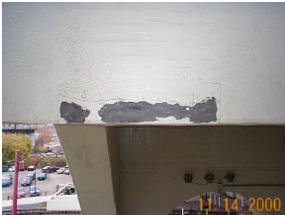
Photo 29 – Span 12, Floorbeam 4, South Bay dcp00245jpg
