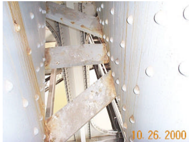
Photo 49 - South Arch L4-L5
