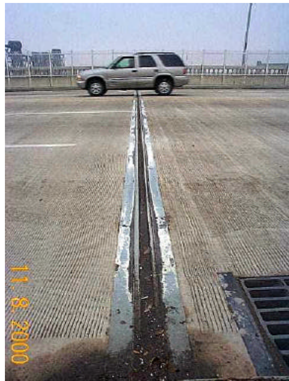
Photo 20 – Expansion Joint dcp00202.jpg
