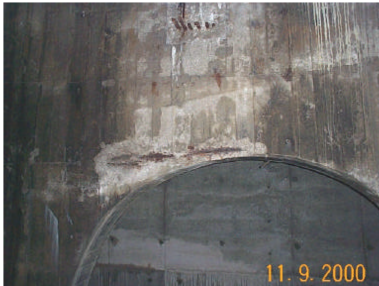
Photo 65 – Pier 3 North Interior Bay
