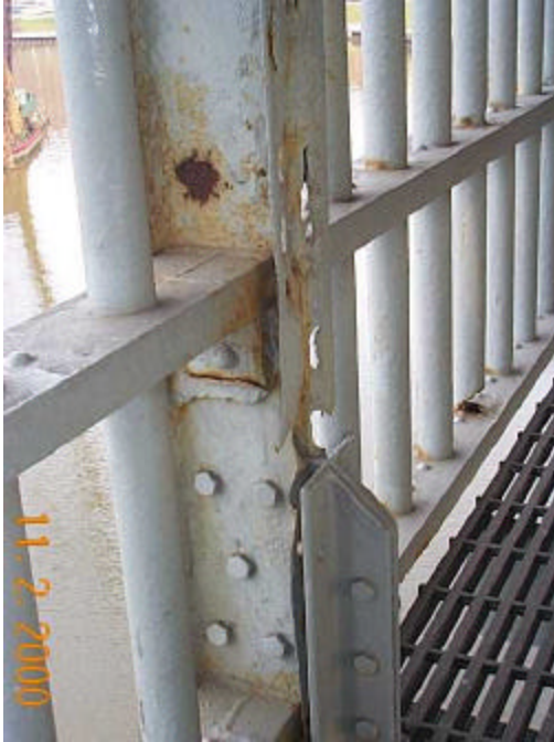
Photo 14 – Holed through exterior railing posts dcp00125.jpg
