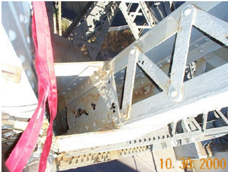
Photo 46 - South Arch at panel point L2
