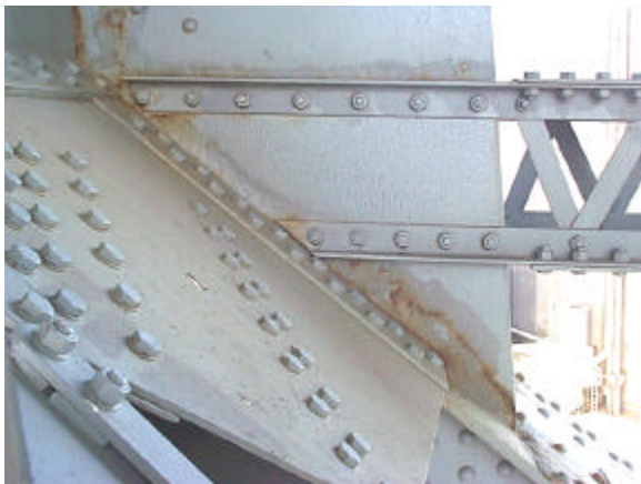
Photo 50a - South Arch North Gusset Plate at L2' dcp00329.jpg
