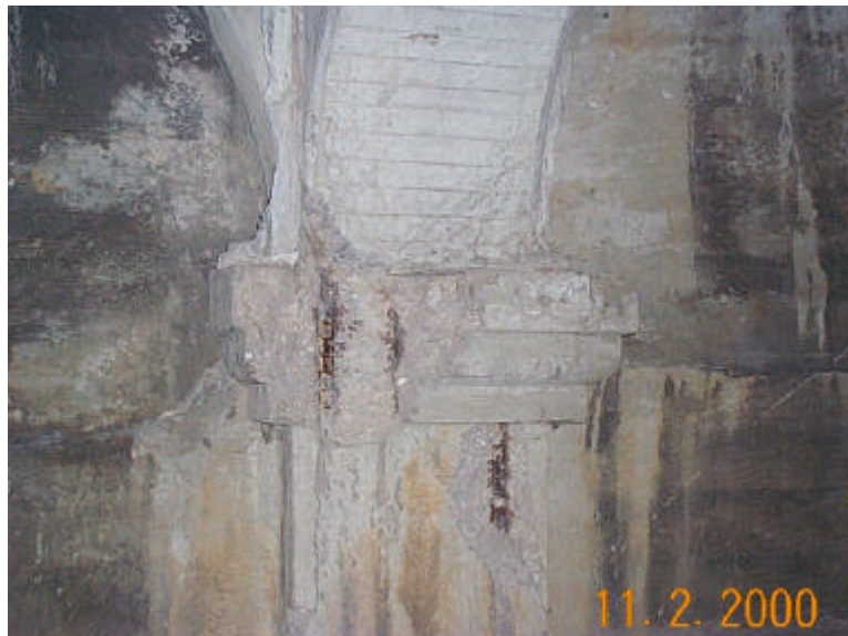
Photo 37 – Span 1A, North Exterior Column 5 dcp00116.jpg
