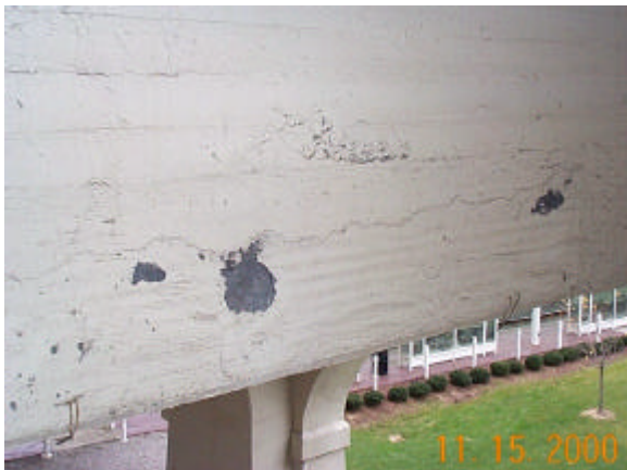
Photo 30 – Span 12, Floorbeam 5, Center Bay dcp00251jpg
