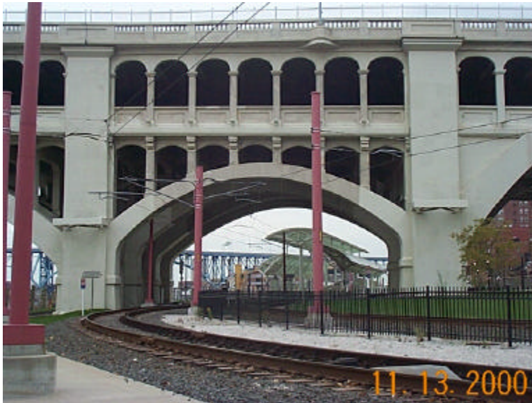
Photo 21 – Typical Concrete Approach, Span 11 dcp00238.jpg
