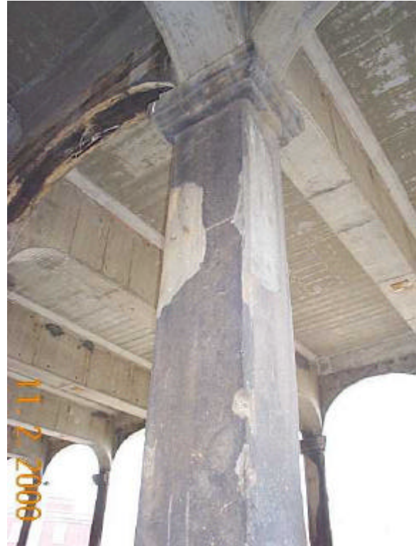
Photo 34 – Span 2, North Int. Column 11 dcp00132.jpg
