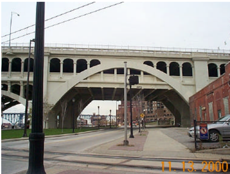
Photo 22 – Concrete Encased Steel Approach, Spans 12 dcp00237.jpg
