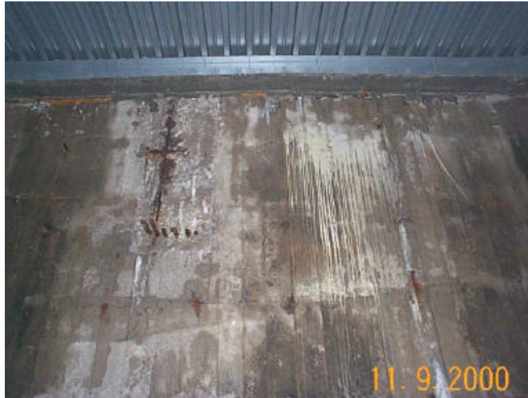
Photo 64 – Pier 3 North Interior Bay
