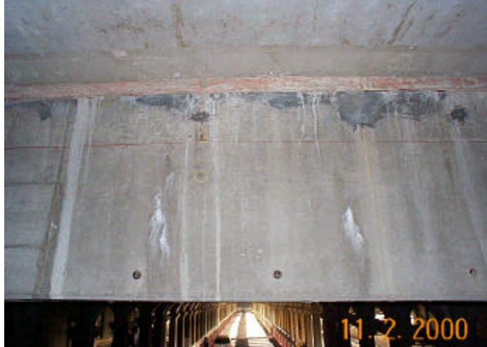
Photo 25 - Span 1A, Floorbeam 4, Center Bay dcp00113.jpg
