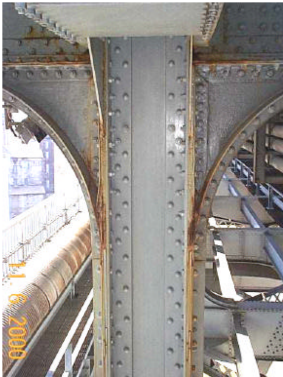
Photo 51 - South Arch at panel point 1'
