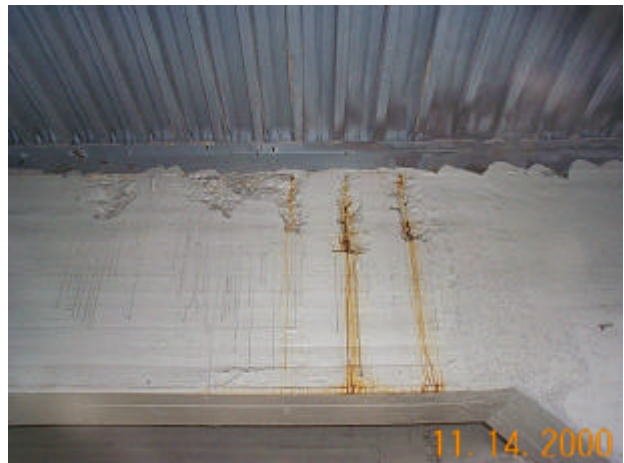
Photo 27 – Span 10, Floorbeam 5, South Bay dcp00240.jpg
