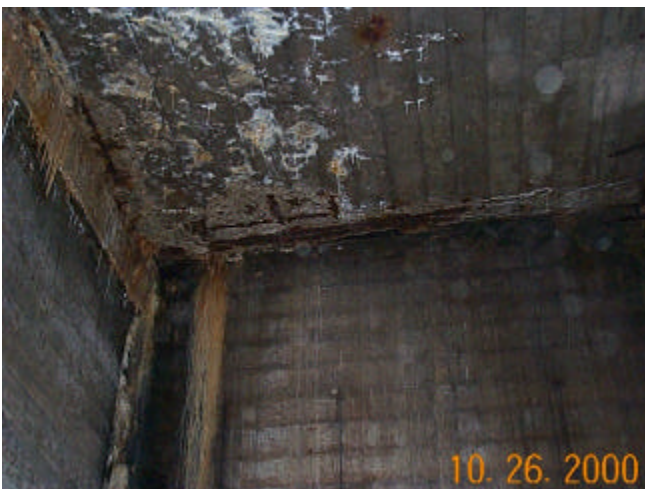
Photo 69 – North Cell, Roof Slab (1 st cell from the West end)
