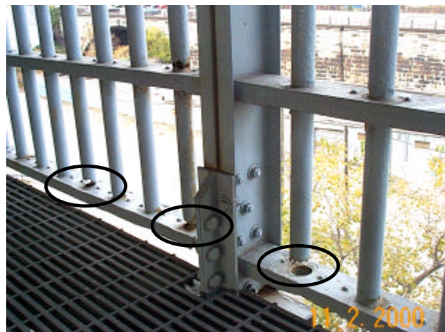
Photo 13 – Holed through vertical tubular rails dcp00123.jpg
