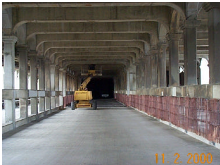
Photo 2 – Lower Deck, Center Bay
