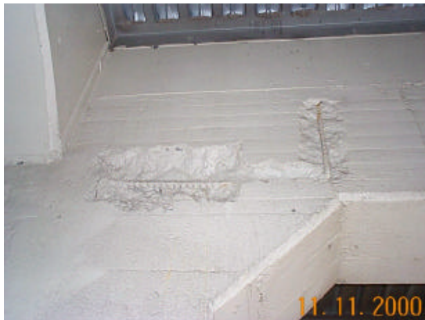
Photo 26 – Span 5, Floorbeam 2, South Bay dcp00226.jpg
