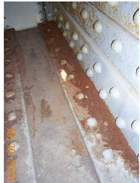
Photo 45 – Debris and Blast Material
