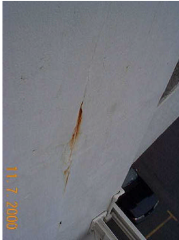
Photo 66 – Pier 9 North Face
