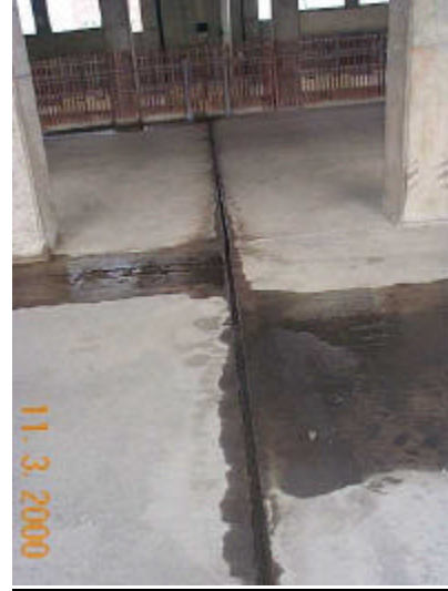
Photo 11 – Lower Deck Compression Joints dcp00146.jpg
