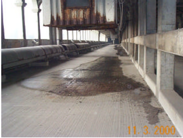
Photo 10 – Lower Deck, South Bay dcp143.jpg
