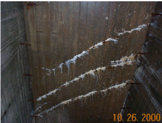
Photo 68 – South Cell, Roof Slab (1 st cell from the West end)
