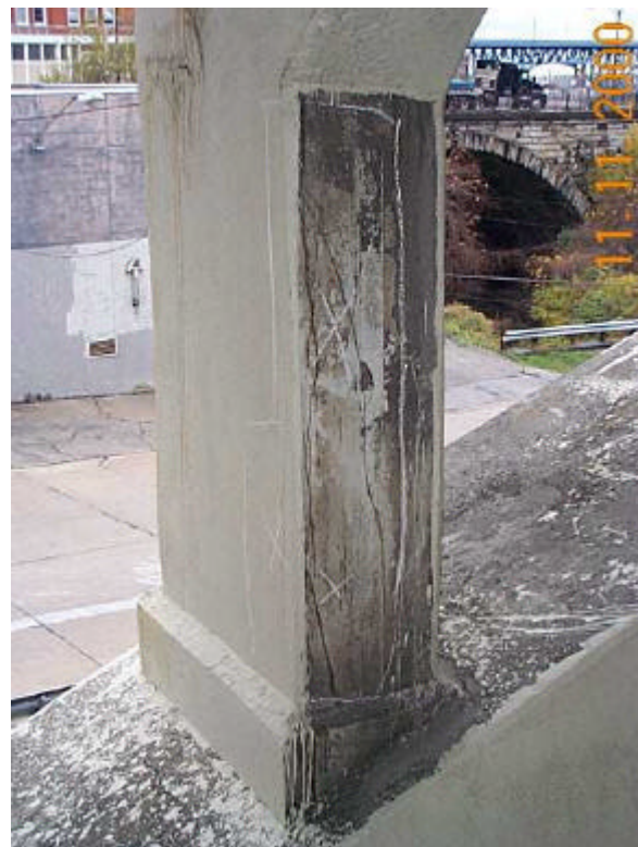
Photo 41 – North Exterior Column 4, Span 2
