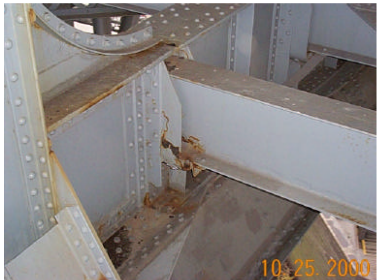
Photo 56 - Lower Deck Stringer 10 at panel point 3'
