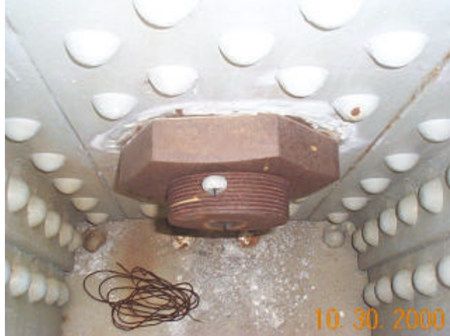
Photo 48 - North Arch Bottom Chord L11'
