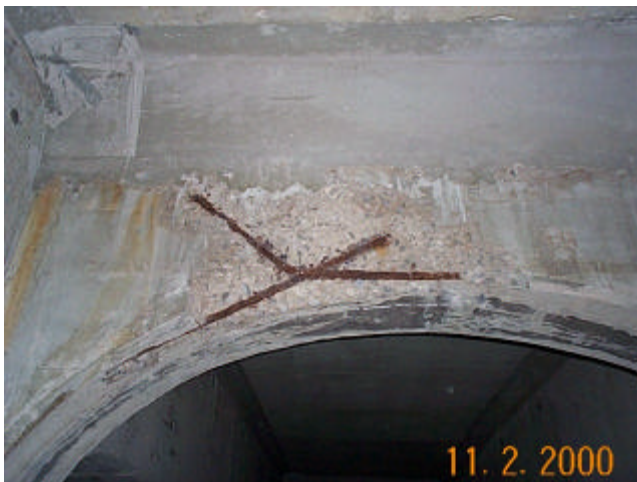
Photo 32 – Span 1A, North Interior Jack Arch between FB 6 & 7
