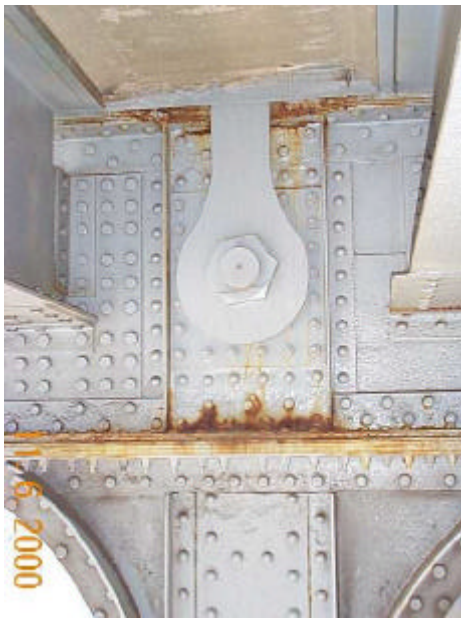
Photo 53 - Upper Deck Floorbeam at 7', South Arch dcp00158.jpg
