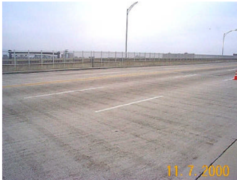
Photo 1 – General Upper Deck
