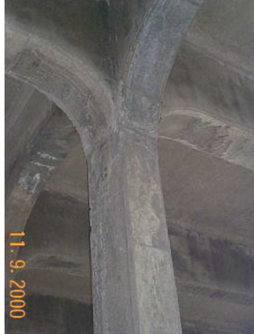
Photo 36 – Span 3, North Interior Col. 13 dcp00212.jpg
