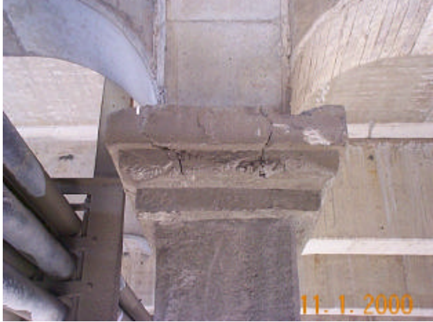
Photo 35 – Span 1 South Interior Column 7 dcp00091.jpg
