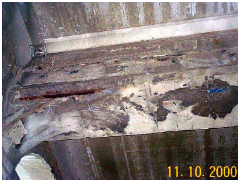
Photo 24 – Span 2, Floorbeam 8, South Bay (original)
