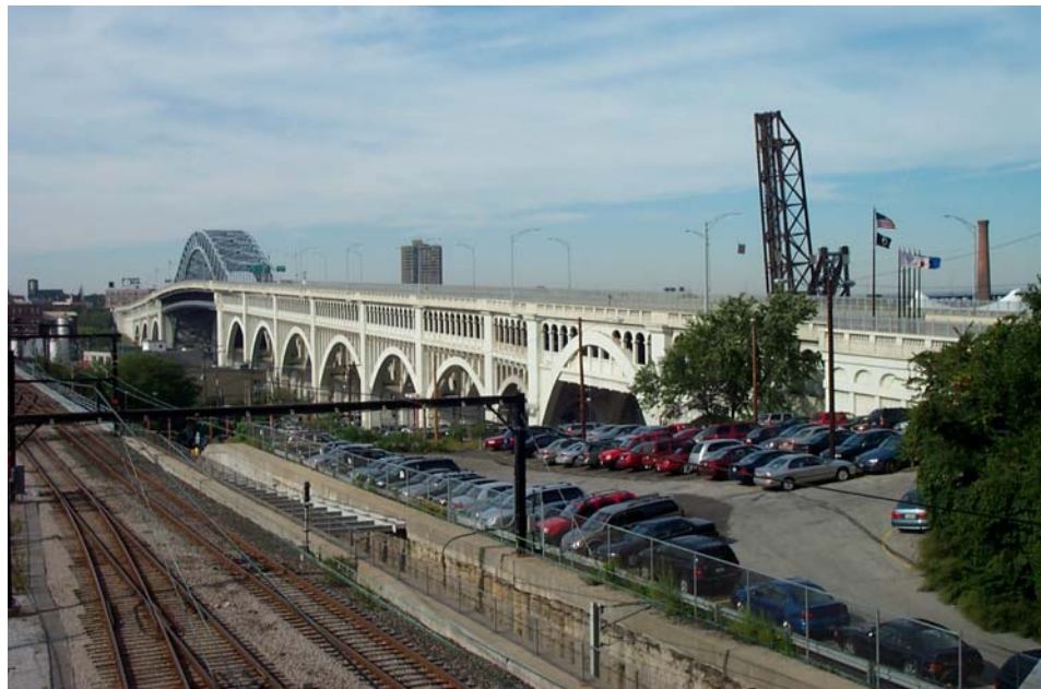
Photo 1. South elevation view looking west.
