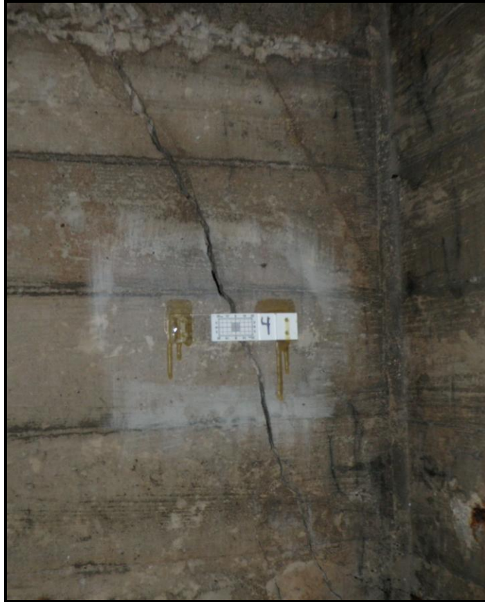
Photo 52: Typical Crack Monitor Installed on a Crack in the Cellular Construction
