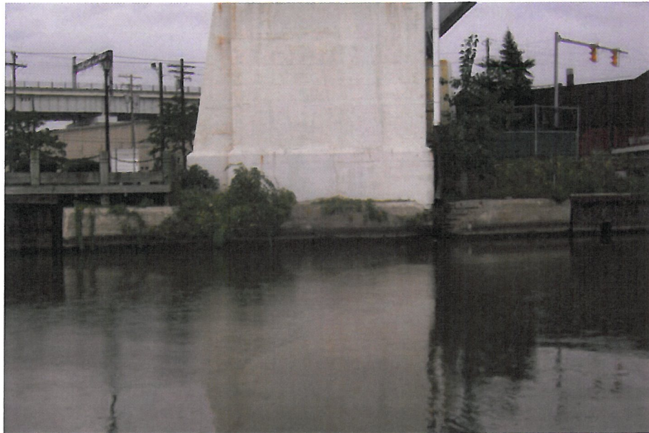
Photo 7 – Facing Southeast. North face of Pier 4 with concrete cap and adjacent steel sheet pile walls.
