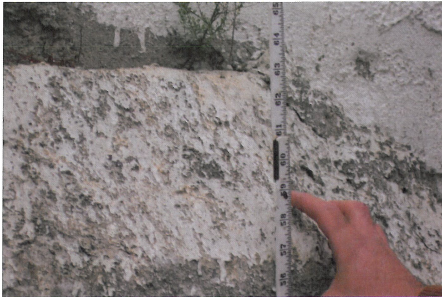
Photo 11 – Facing South. Hydrographic Reference Point Top of wall concrete cap next to Pier 4 is 5.25 feet above the water surface.
