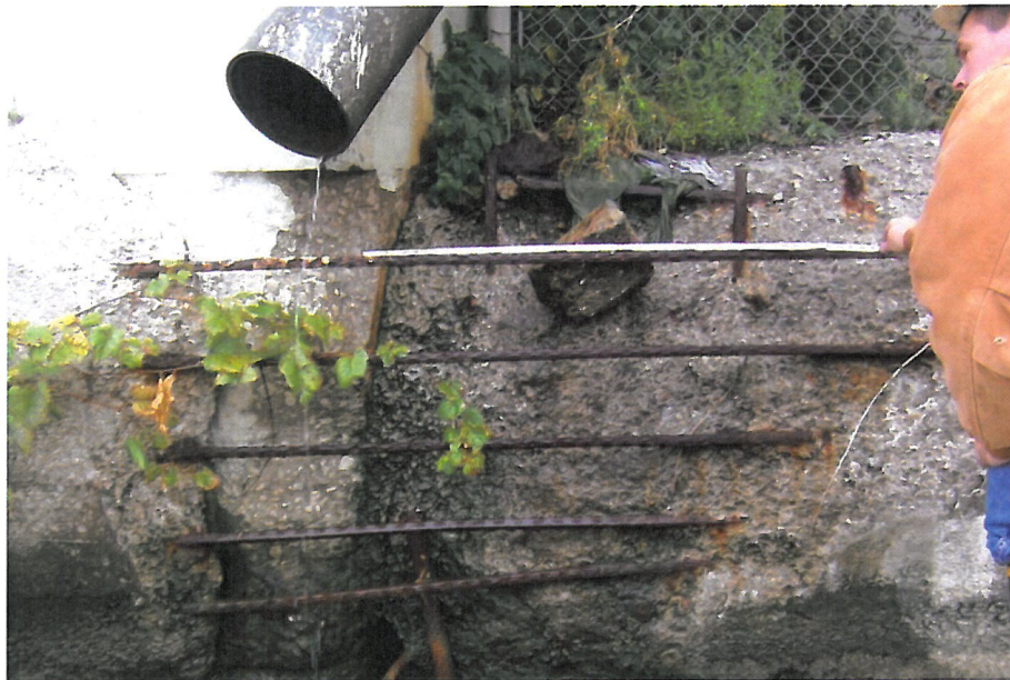
Photo 8 – Facing East. Southwest corner of Pier 4 shown behind the deteriorated concrete cap and exposed rebar .
