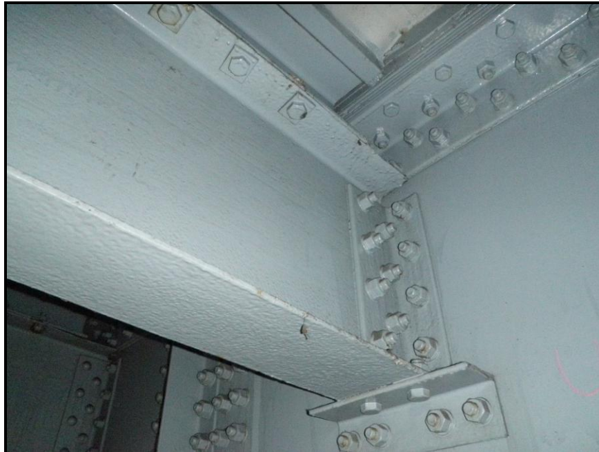
Photo 13: Old Pitting in Upper Deck Stringers
