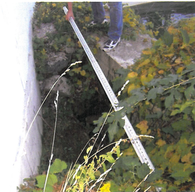
Photo 10 – Facing Southwest. Sinkhole between Pier 4 and wall concrete cap. Sinkhole is 4 feet wide by 8.5 feet long by 5 feet deep with the water surface visible.
