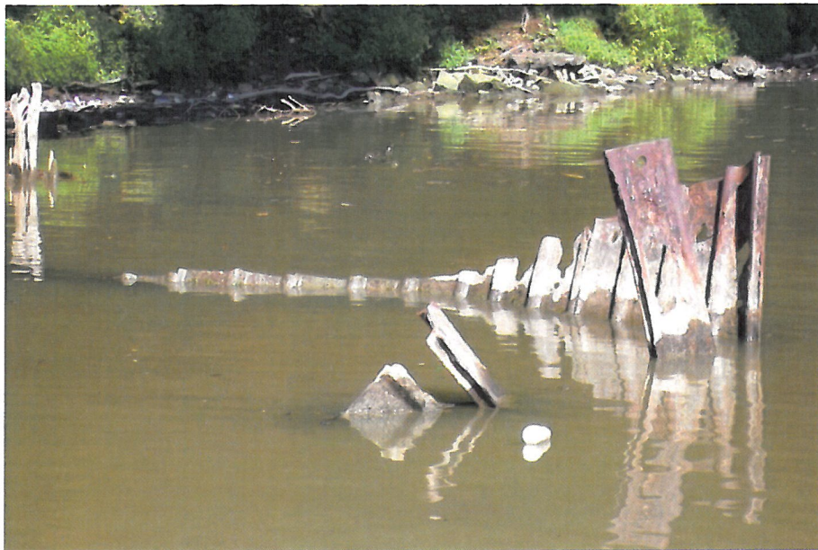
Photo 12 – Facing North. Steel Sheet pile Wall on the north side of Pier 3.
