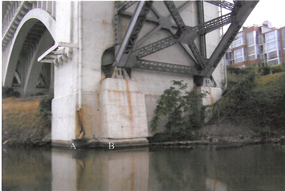
Photo 5 – Facing West. East face of Pier 3. Note Scupper Pipe disconnected allowing water to run down the east face of the Pier 3.
