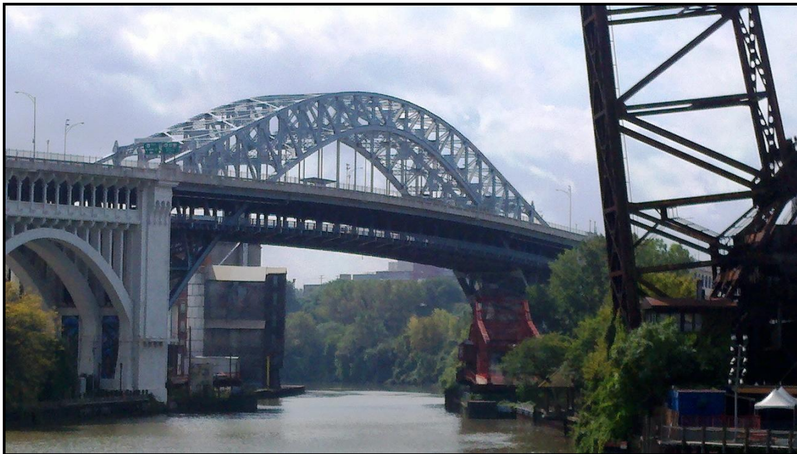
Detroit-Superior Bridge over the Cuyahoga River - South Elevation View of Span 4
