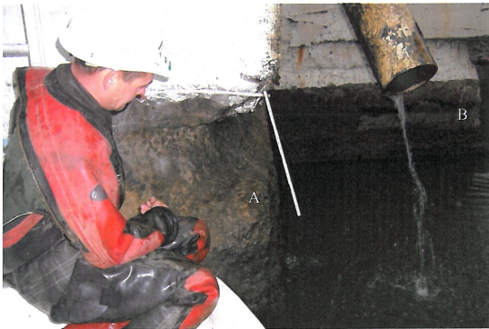
Photo 6 – Facing North. Southeast corner of Pier 3. Note the Scaling and Spalling of the concrete at the construction joint.
