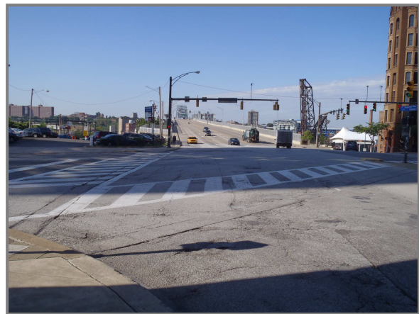
Photo 38 – View looking west from the East Approach
