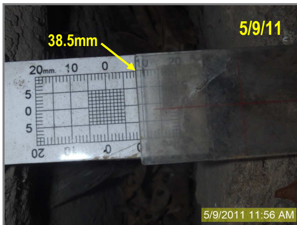
Photo 33 – May 9, 2011 South Tower B gauge reading.
