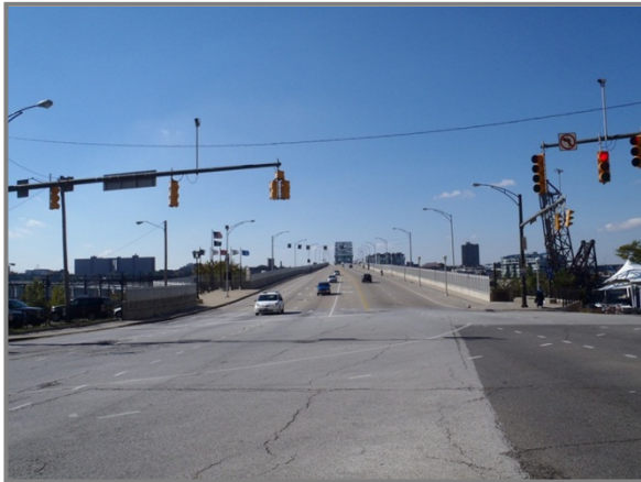
Photo 52 – General view looking toward the structure from the East Approach.
