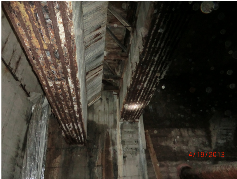
Lower deck floor beams at East Abutment.
