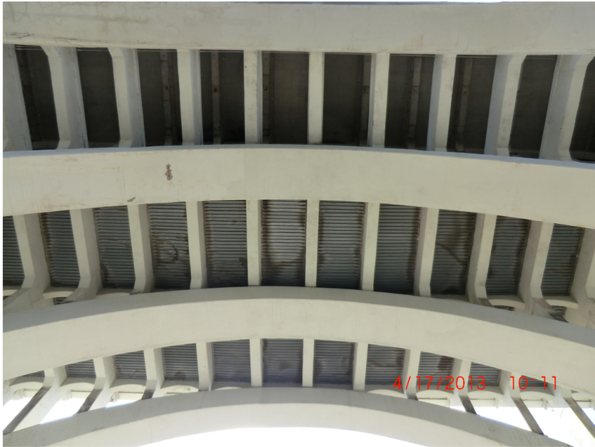
Span 5 arches and lower deck floorbeams
