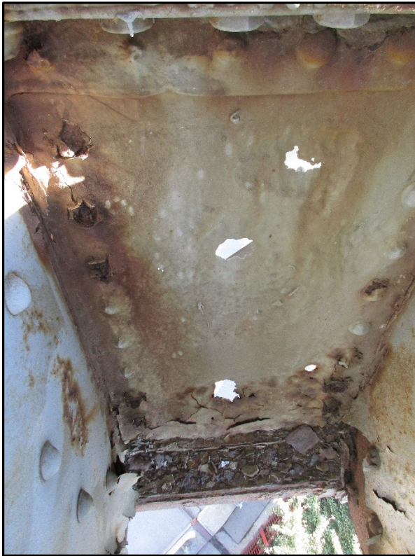
Photo 34 – Common Perforations of Lower Chord Diaphragm.
