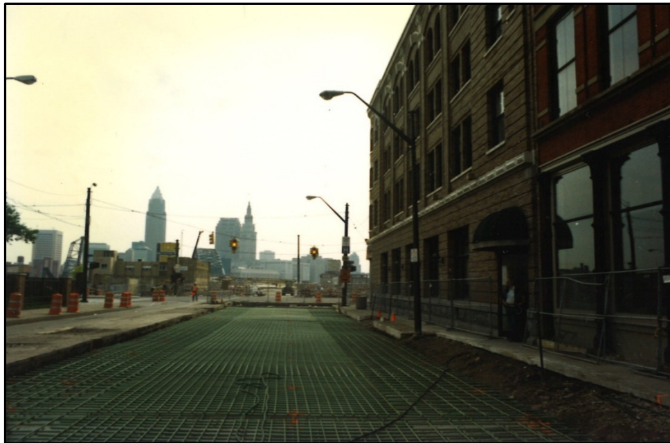
Photo 4 - Construction of Detroit Avenue Tunnel Supplemental Roof Slab, Looking East, 1996.
