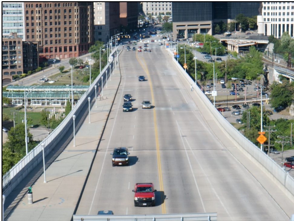
Photo 2– East Approach Spans Deck, Looking East.
