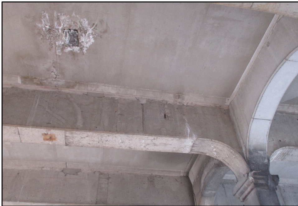
Photo 8 – Full Depth Upper Deck Floor Patch, Span 9.
