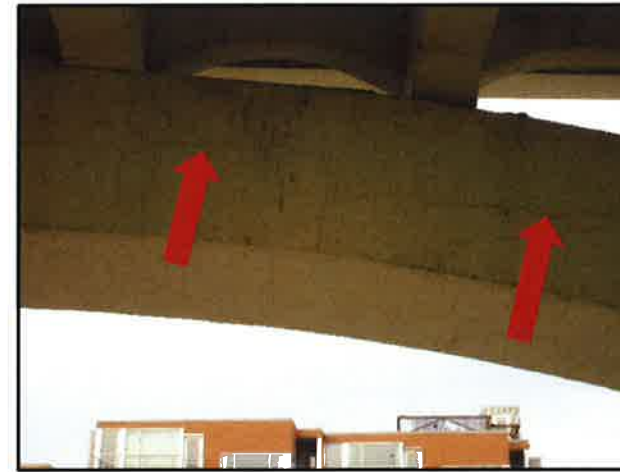
Photo B4 - Panels 11 & 12.
