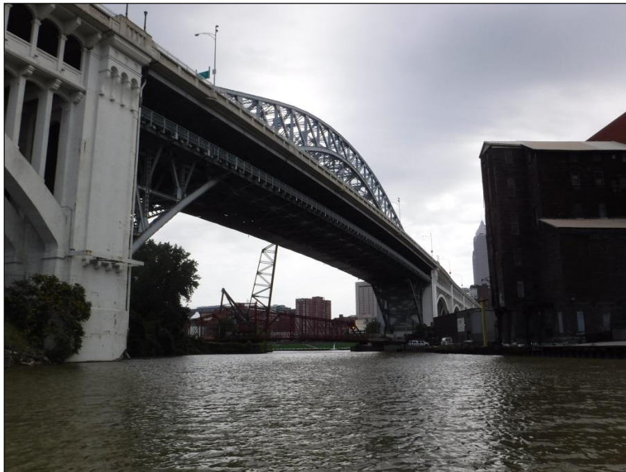
(South Elevation of Bridge)
