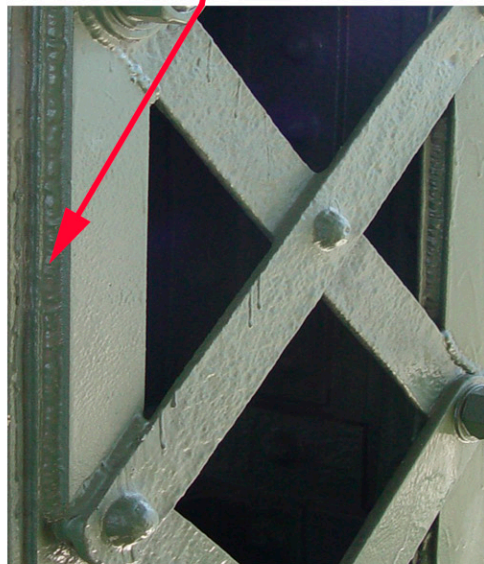
WELDED PLATE TO VERTICAL THIS IS TYPICAL TO SEVERAL LOCATIONS.
