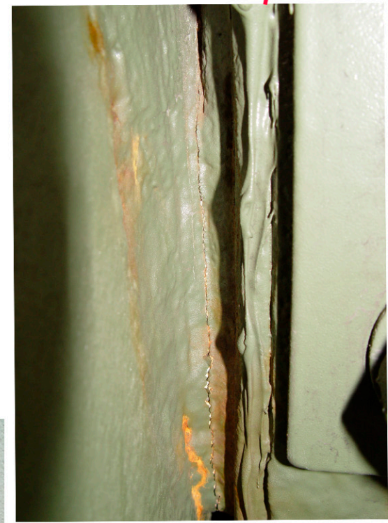
CLOSE UP OF ABOVE PHOTO.
