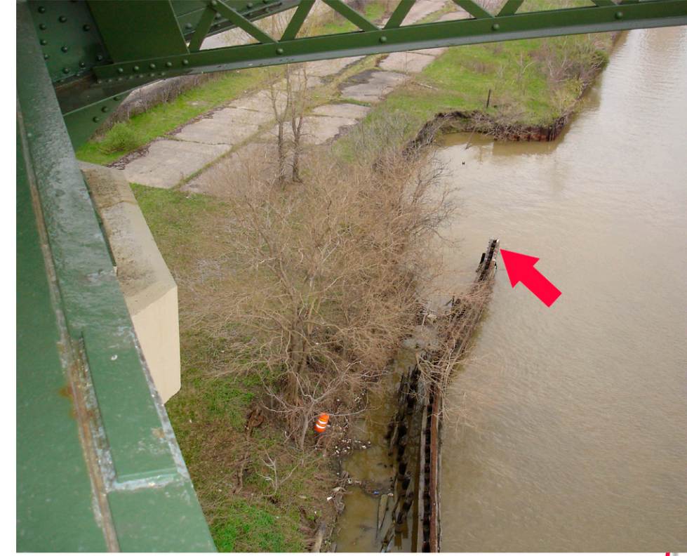
PHOTO SHOWS HOW RIVER FLOWS INTO AND ERODING THE WEST BANK. RED ARROW SHOWS THE END OF DOWN RIVER FENDER.
