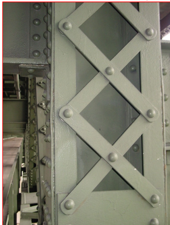
Typical good condition of paint after rehabilitation. Most members, like U8-L8 shown here, have some previous pack rust that has been cleaned and painted over and is not currently active.
