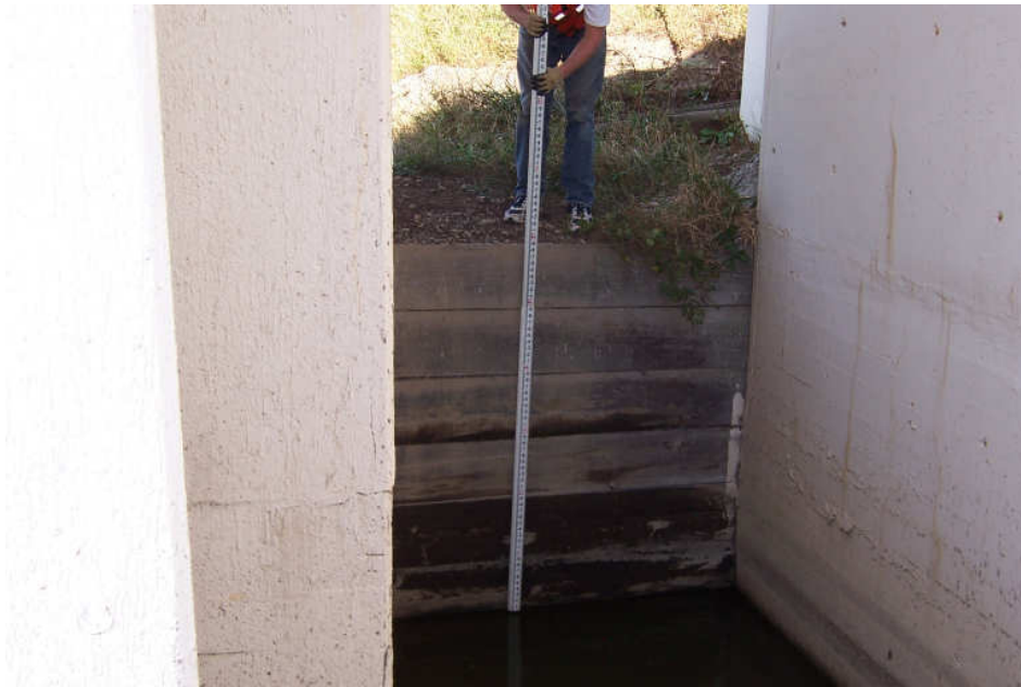
Photo 10 – Facing West. Hydrographic Reference Point Timber Retaining Wall 5.9 feet above water surface.
