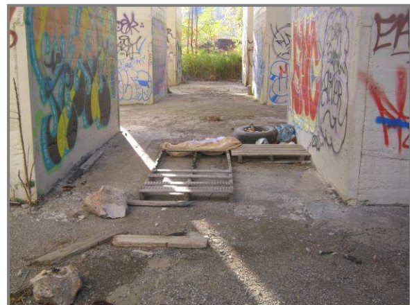
Photo 68– Old mattress and trash piles at Pier 7.
