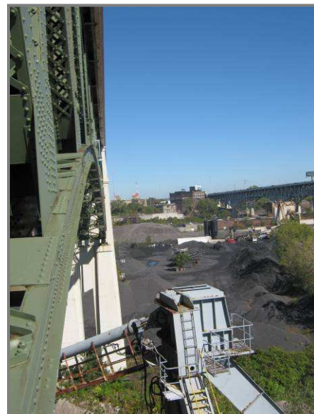
Photo 66– Vertical clearance between truss and top of vessel under Truss D.
