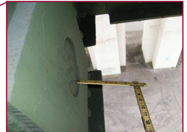
The lower chord sliding pin at CL100 is not bearing fully on the outermost pin plate.
