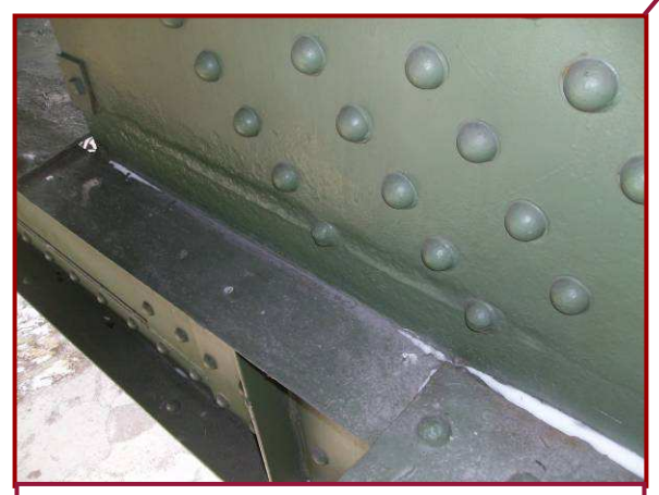
Up to 1/8" pitting is present on the south face of gusset plate AL129S along the bottom row of rivets.
