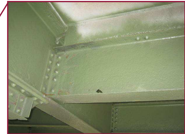
Stringer 2 between AU117 and AU118 exhibits advanced section loss with less than 1/8" section remaining for the full height of the web near AU118. A 4" diameter hole is present in the web at the flange.
