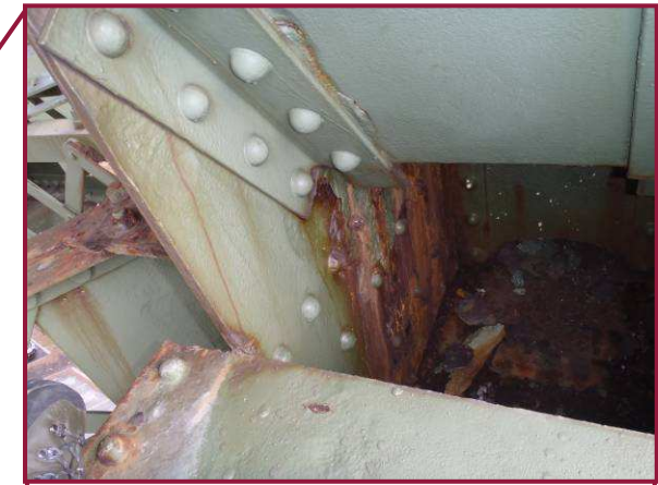
South face of DL113N at west end of plate.
