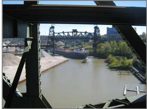
Photo 64– Bend upstream (south) of the bridge crossing.
