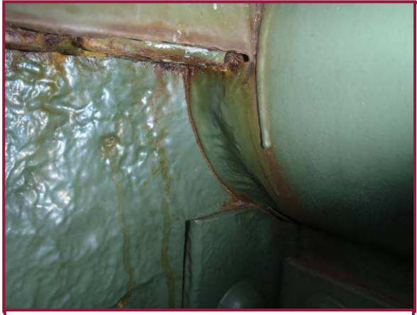
The bearing pin at AL12 exhibits 3/16" deep loss along the circumference adjacent to the pin plates. Additionally, the innermost pin plates exhibit 1/8" deep pitting throughout the interior face adjacent to the pin.
