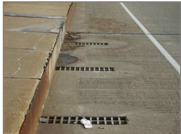
Photo 7 – Typical roadway drain with minor water pooling around drain.
