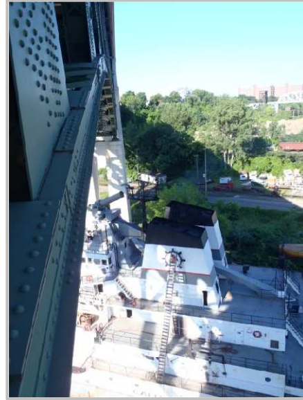
Photo 57 – Vertical clearance between structure and top of vessel under Truss A.
