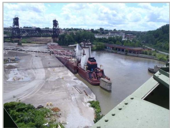
Photo 56 – General view upstream (south) of bridge crossing, showing bend in channel.
