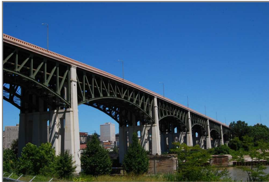
Figure 1 – CUY-10-1613 elevation looking northeast
