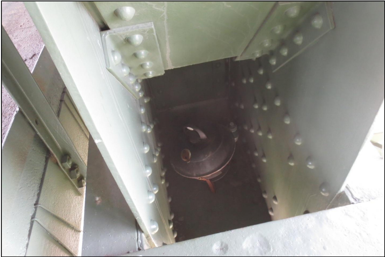
Photo 49 – Grill Hidden within Lower Chord Panel Point, Span 10.
