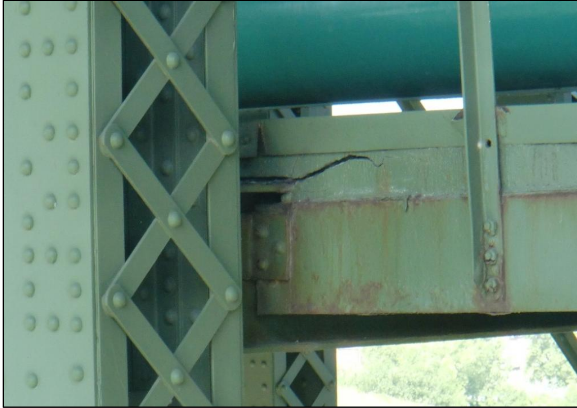
Photo 12 - Maintenance Deck at Floor Beam 17, Span 11.
