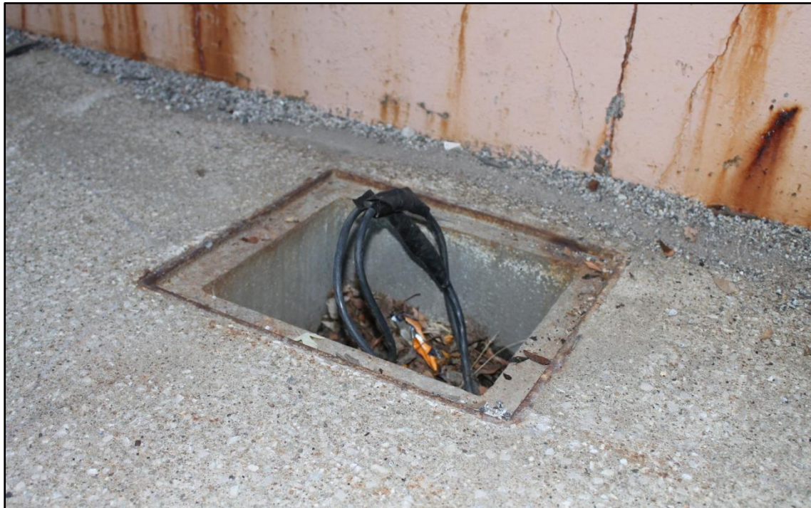
Photo 16 – Open Pull Box, South Sidewalk, Span 13.
