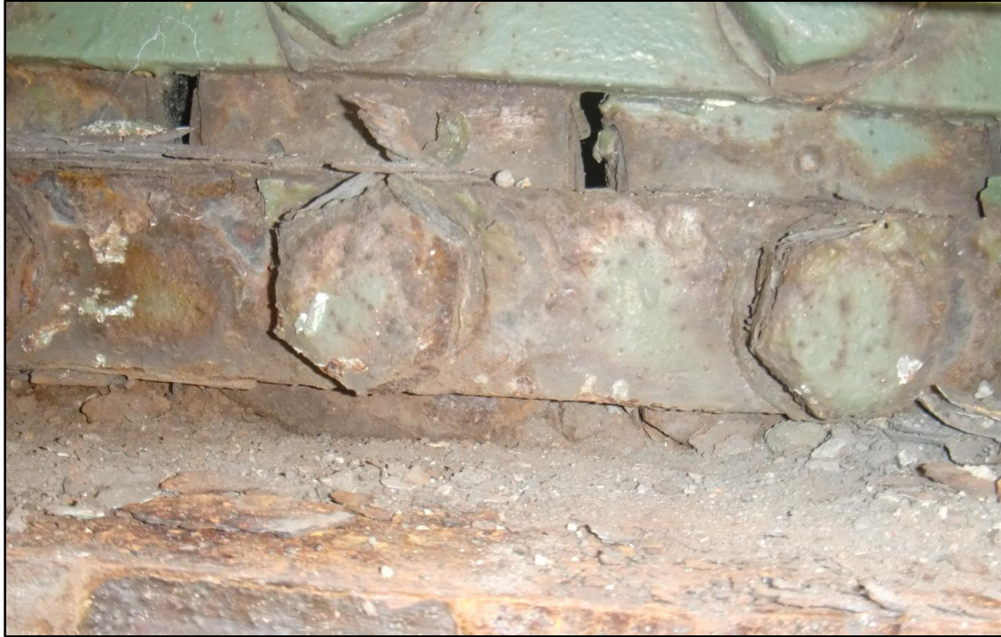
Photo 33 – Typical Debris within Expansion Rollers.
