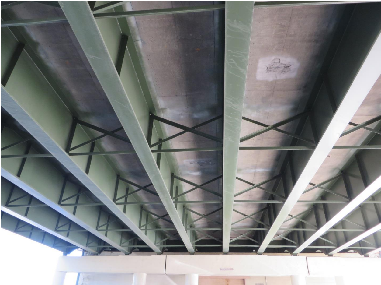
Beams and cross frames in the west approach
