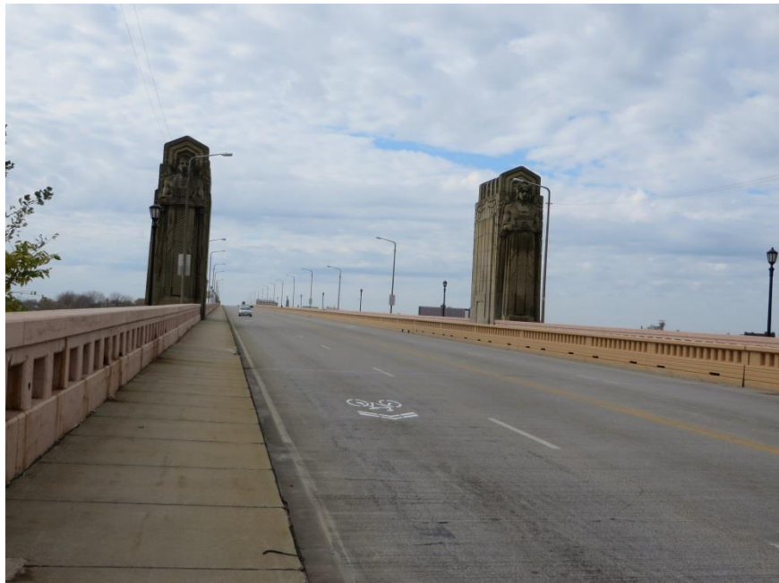
East approach guardrail
