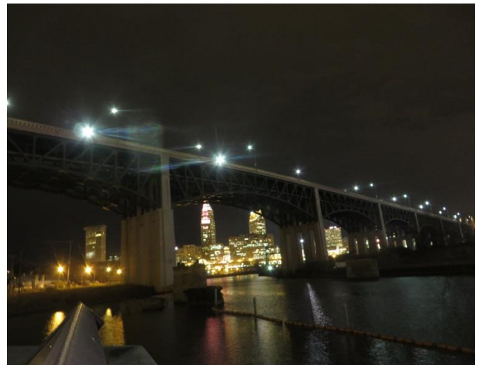
Navigation Lights not working
