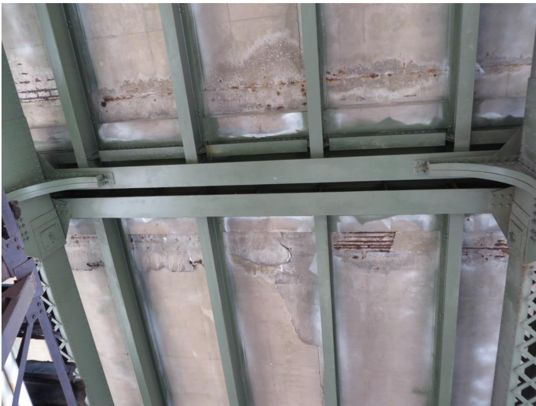
Typical slab condition adjacent to expansion joints
