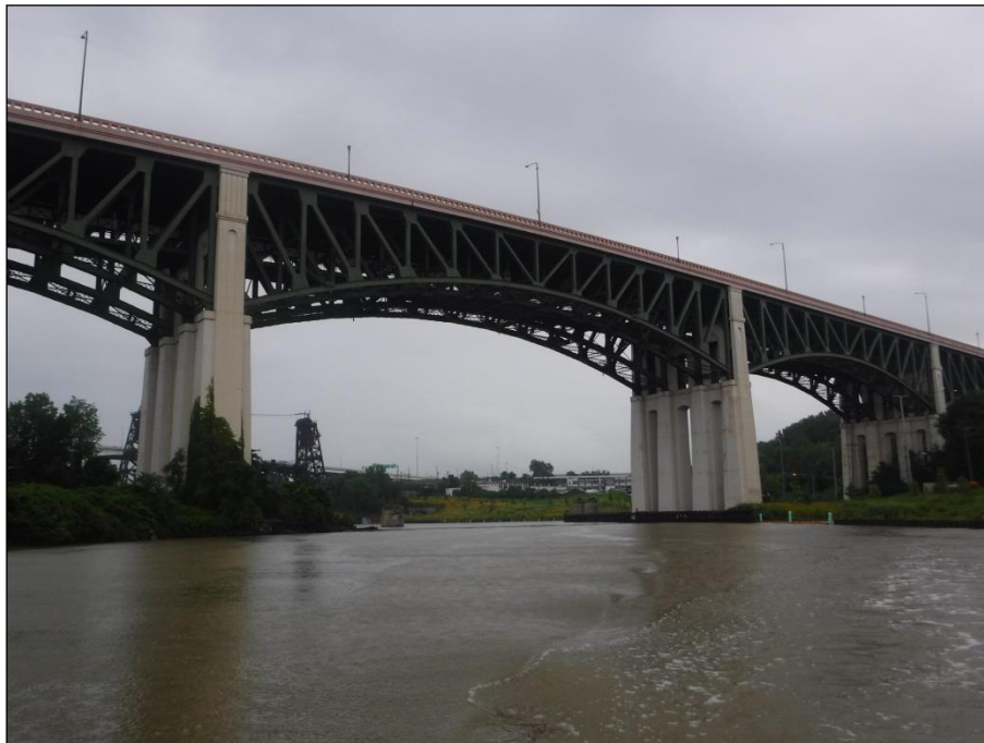
(North Elevation of Bridge)
