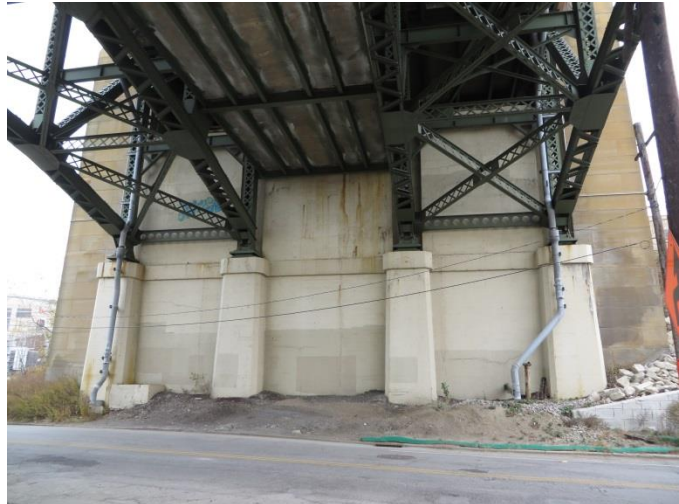
East abutment face
