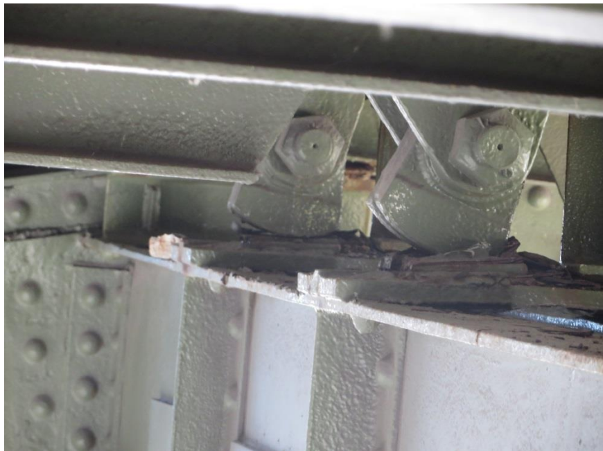
Utility deck bearing condition from C-S03-LC-13
