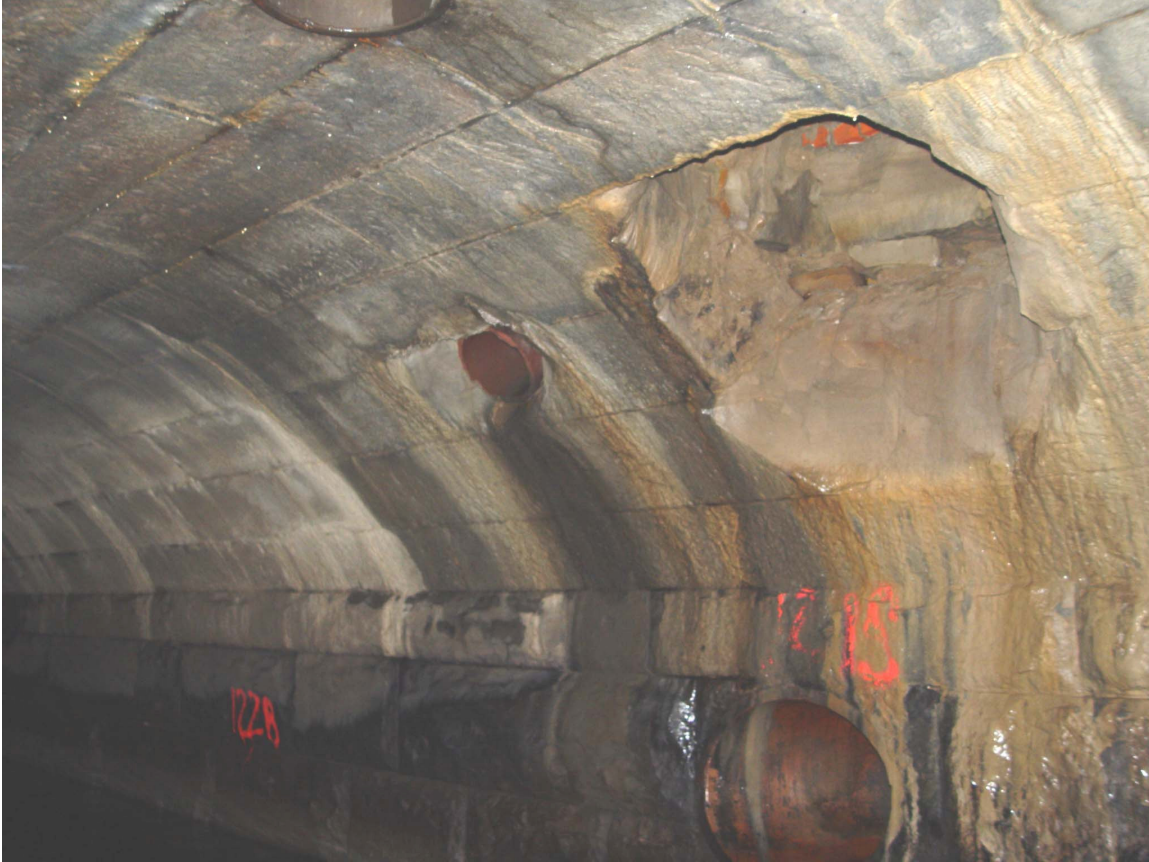
Photo 1. Stones have been removed from arch to a connect catch basin.
