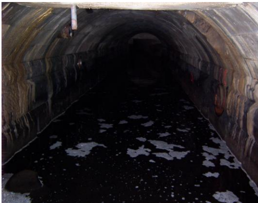
General View of Stone Arch Culvert
