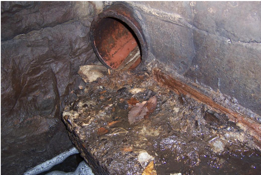
Photo 12 – Facing East. 106' north of the cemetery entry manhole. 12" diameter inlet pipe in the southeast corner of the stone arch culvert
