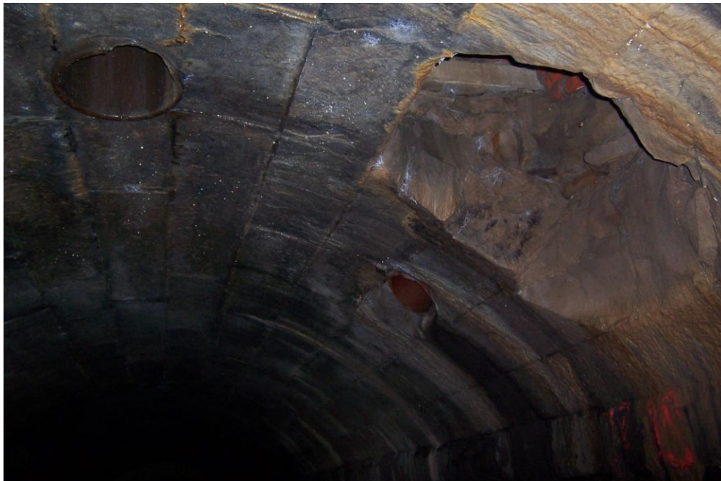
Photo 14 – Facing Northeast. 122’ north of the cemetery entry manhole. 12” diameter pipe in the east wall and 18” diameter pipe in the crown.
