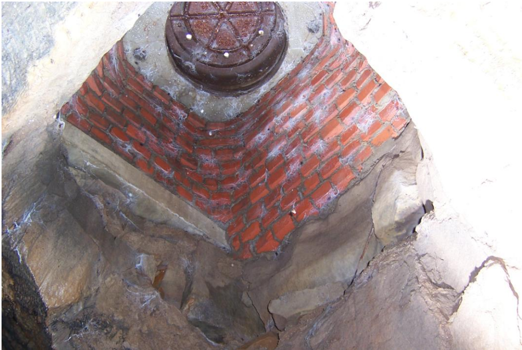
Photo 7 – Facing Northeast at 122’ north of the cemetery entry manhole. Manhole entrance into the stone arch culvert.
