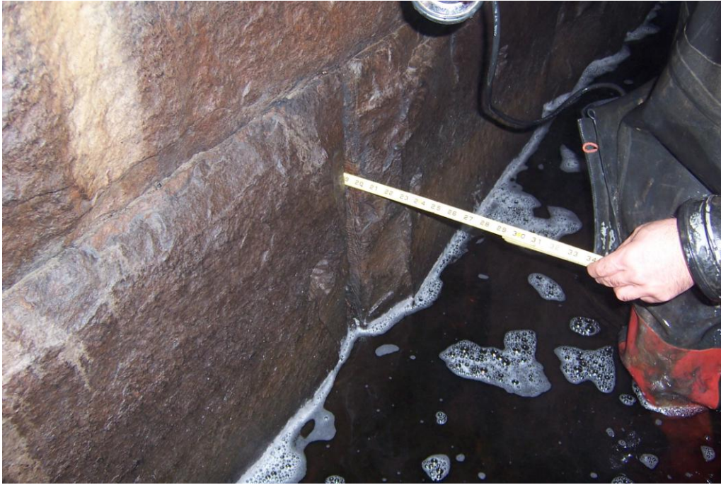
Photo 23 – Facing West. Typical missing mortar along the waterline of the stone arch culvert.
