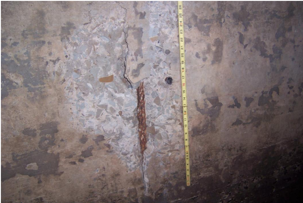
Photo 21 – Facing East. 85' north of the cemetery entry manhole. 30" high x 18" wide x 3" deep spall with exposed reinforcing steel.
