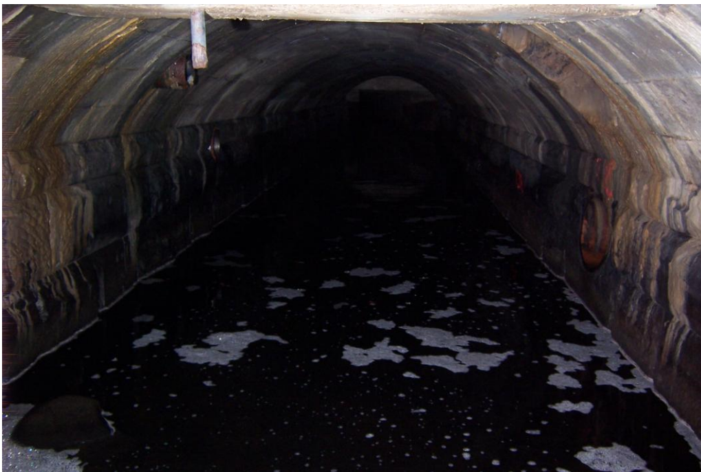
Photo 4 – Facing North. Stone Arch Culvert.
