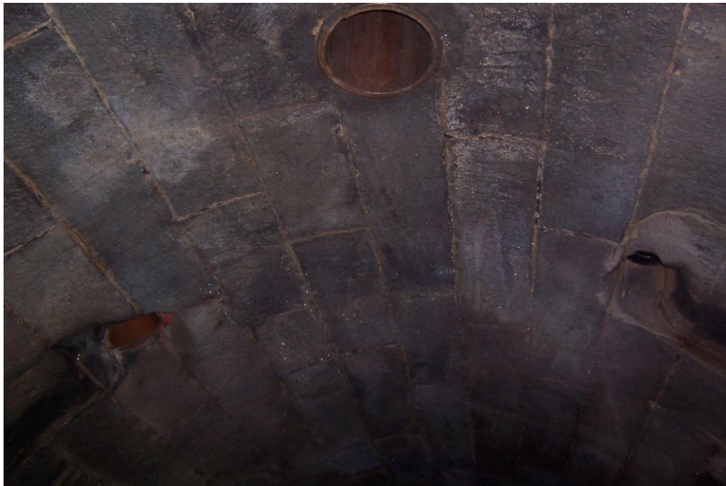
Photo 18 – Facing South. 170' north of the cemetery entry manhole. 12" diameter pipes in the sides and 18" diameter pipe in the top of the stone arch culvert crown.
