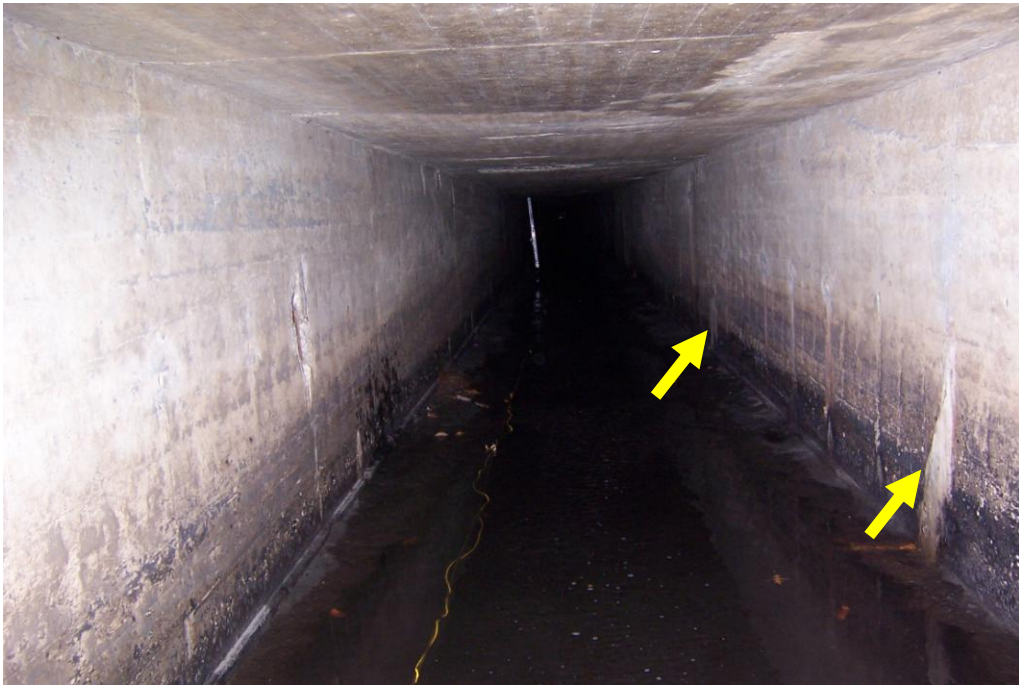
Photo 3 – Facing South. Concrete Box Culvert. Also showing typical hairline wrap-around cracks.
