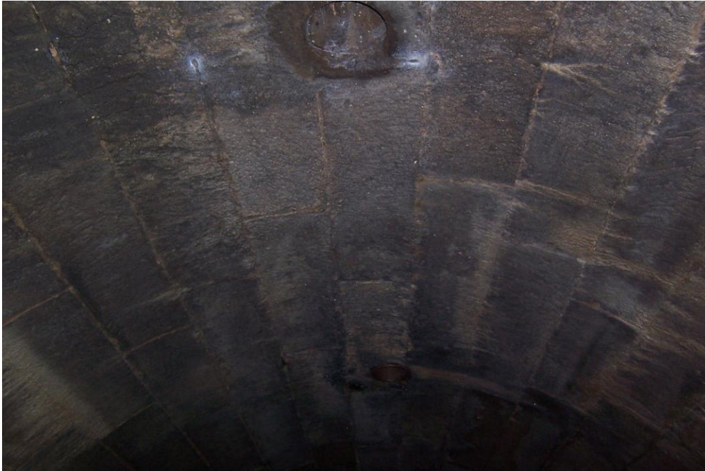
Photo 17 – Facing North. 145' and 155' from the cemetery entry manhole. 12" diameter inlet pipes in the crown of the stone arch culvert.
