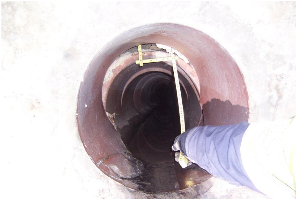
Photo 10 – Facing West. 20’ north of the cemetery entry manhole. 18” diameter inlet pipe with an offset section and exposed fill.
