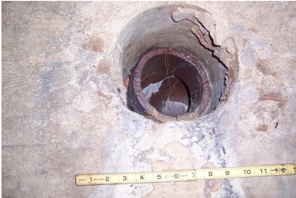
Photo 9 – Facing East. 20’ north of the cemetery entry manhole. 6” diameter inlet pipe with edge spalling.
