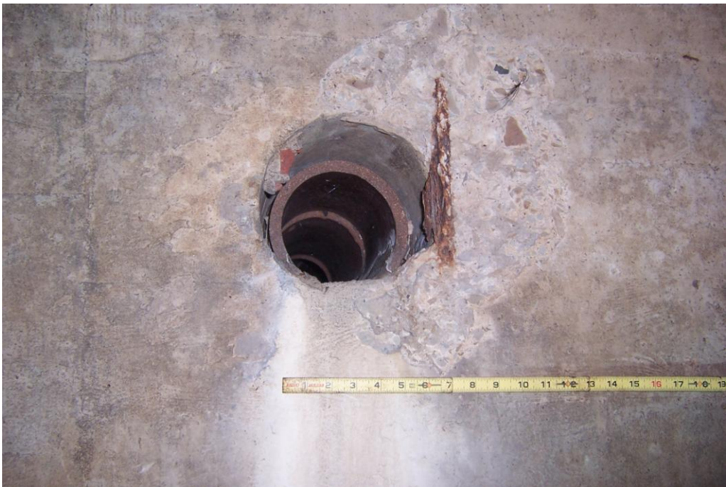
Photo 8 – Facing West. 20’ north of the cemetery entry manhole. 6” diameter inlet pipe with an adjacent 8” wide x 16” high x 1” deep spall with exposed corroded reinforcing steel.
