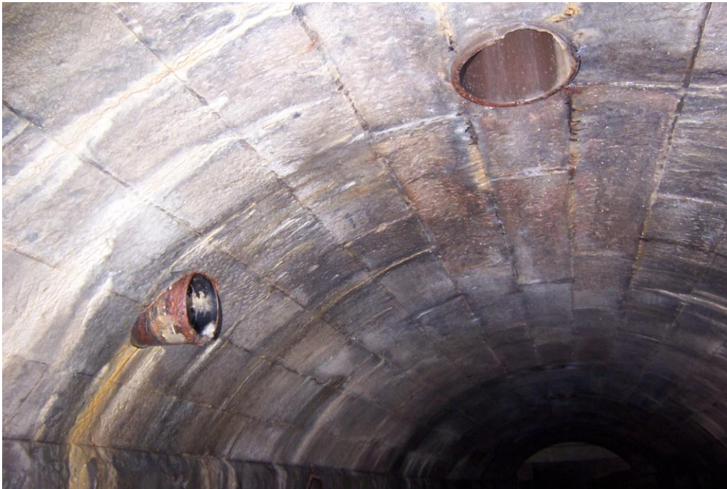
Photo 13 – Facing Northwest. 122’ north of the cemetery entry manhole. 12” diameter pipe in the west wall and 18” diameter pipe in the crown.
