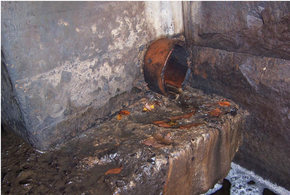
Photo 11 – Facing West. 106' north of the cemetery entry manhole. 12" diameter inlet pipe in the southwest corner of the stone arch culvert.
