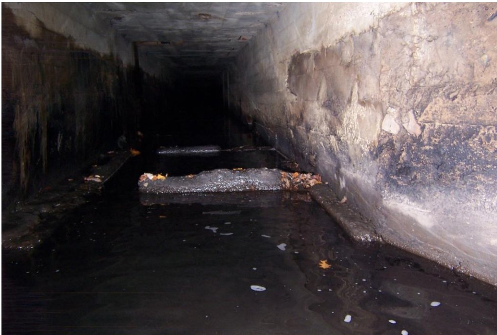
Photo 6 – Facing North. Weir walls along the bottom of the concrete box culvert at the north end of the stone arch culvert.
