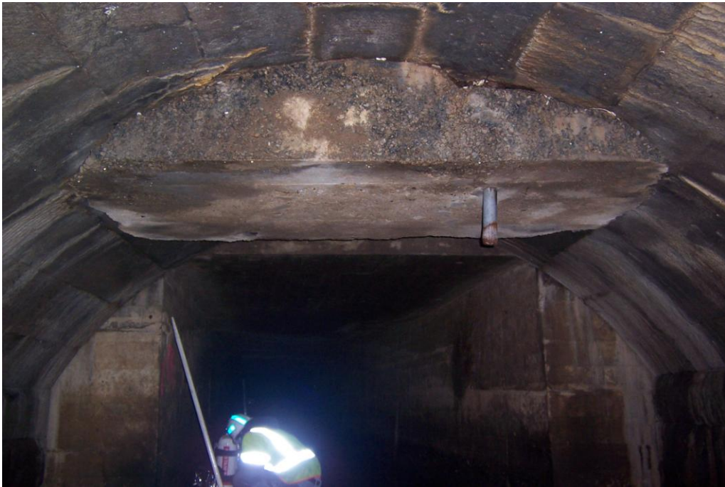
Photo 19 – Facing South. 110’ north of the cemetery entry manhole. Concrete pour at the south end of the stone arch culvert.
