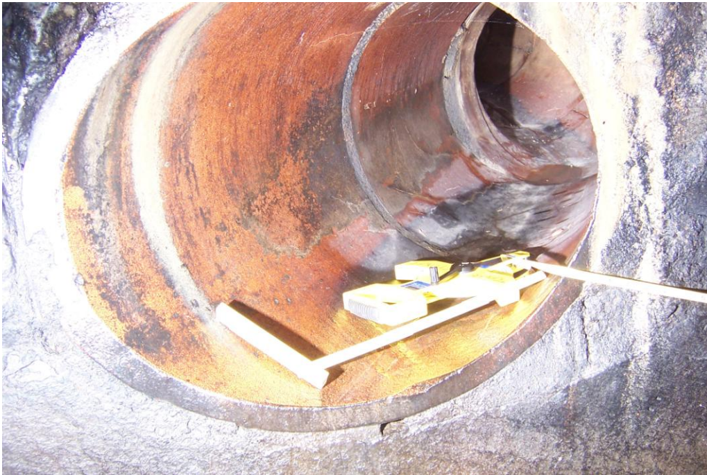
Photo 15 – Facing East. 122’ north of the cemetery entry manhole. 18” diameter inlet pipe in the east wall of the stone arch culvert
