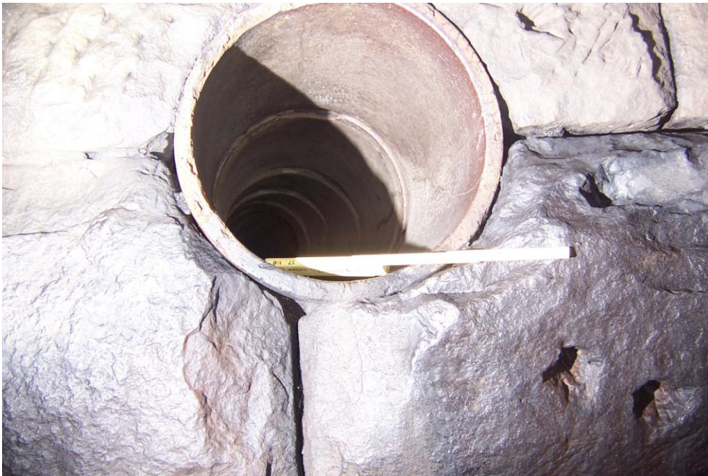
Photo 16 – Facing West. 136’ north of the cemetery entry manhole. 20” diameter inlet pipe in the west wall of the stone arch culvert
