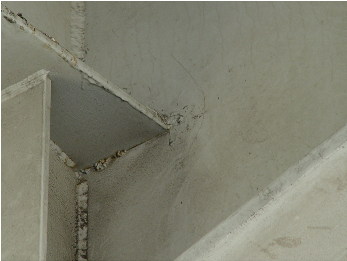
Photo 3. In several locations where a backer bar was not used the weld lacks full penetration between the flange and web plates.
