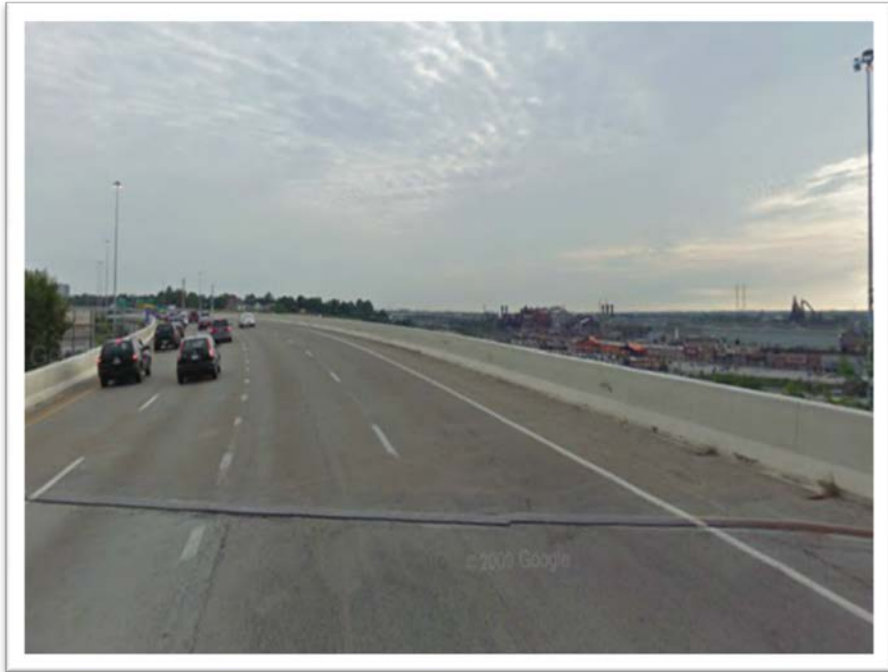
End View Looking South
