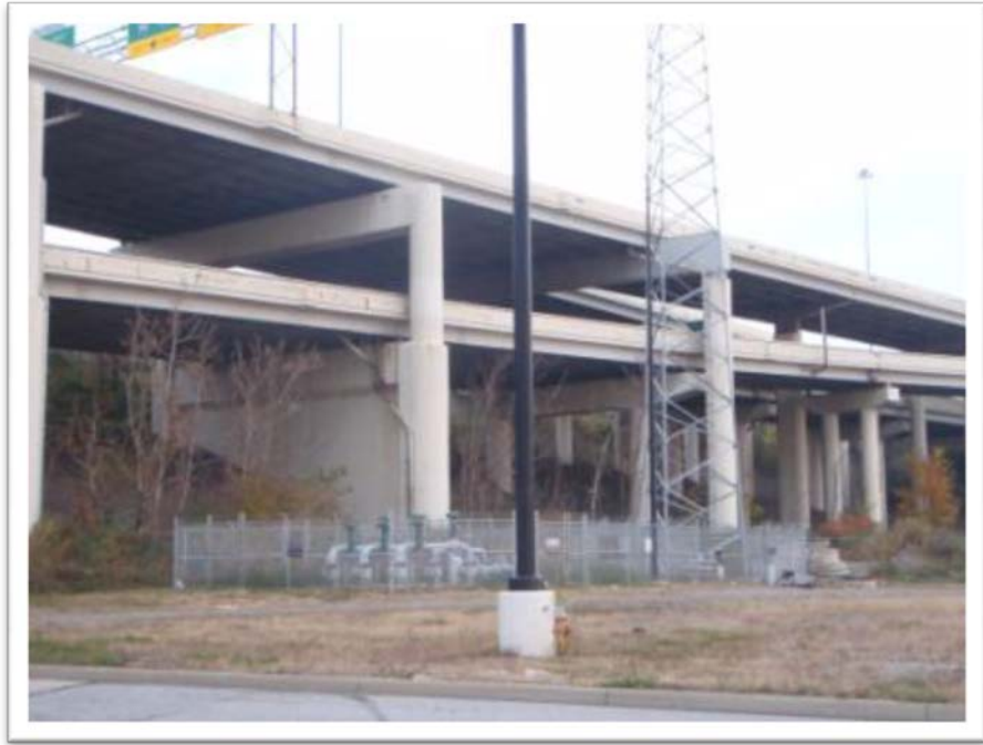
Elevation View Looking West
