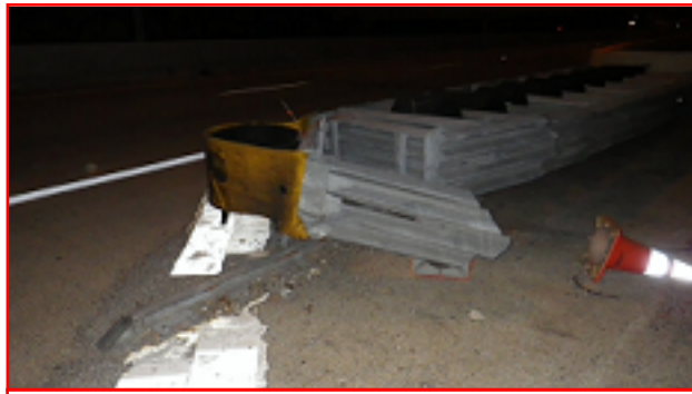
Impact attenuator has been hit by vehicle.
