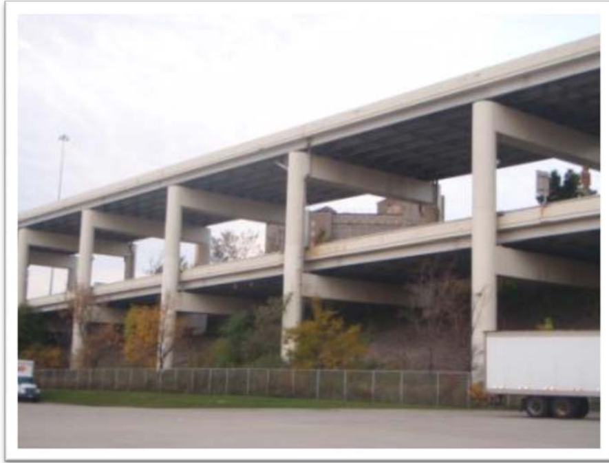
Elevation Looking Southwest
