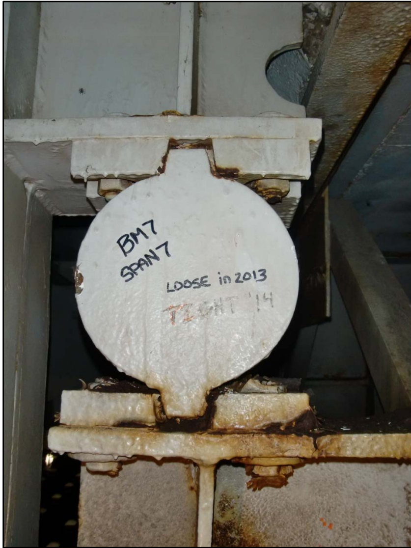
Photo 27 – Now-Tight Hinge at Beam K (7), Span 7.
