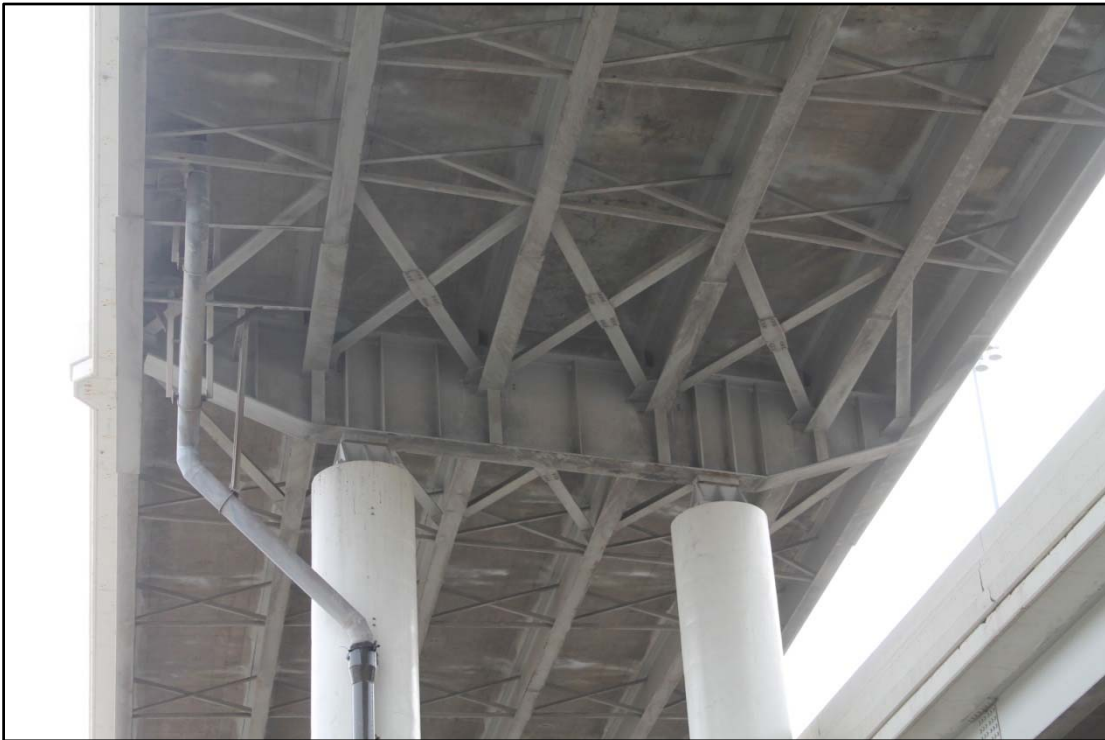
Photo 2- Fracture Critical Steel Pier Cap, Pier 20AE.
