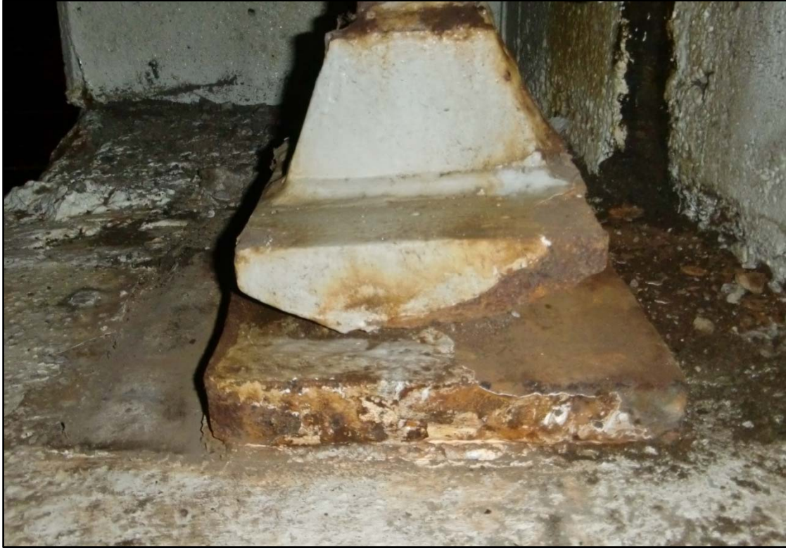
Photo 22 – 3 1/2" Slide of Bearing Plate, Bearing G, North Abutment AE.
