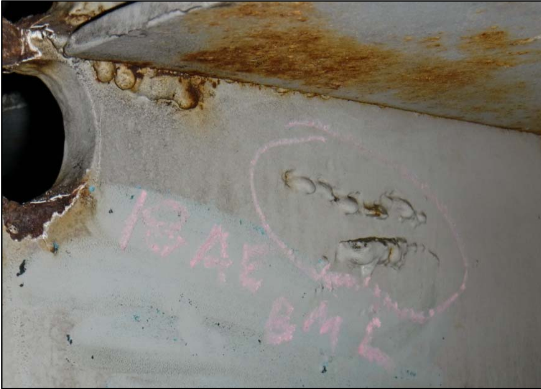
Photo 37 – Weldment on South Web Face, Steel Pier Cap 18AE.
