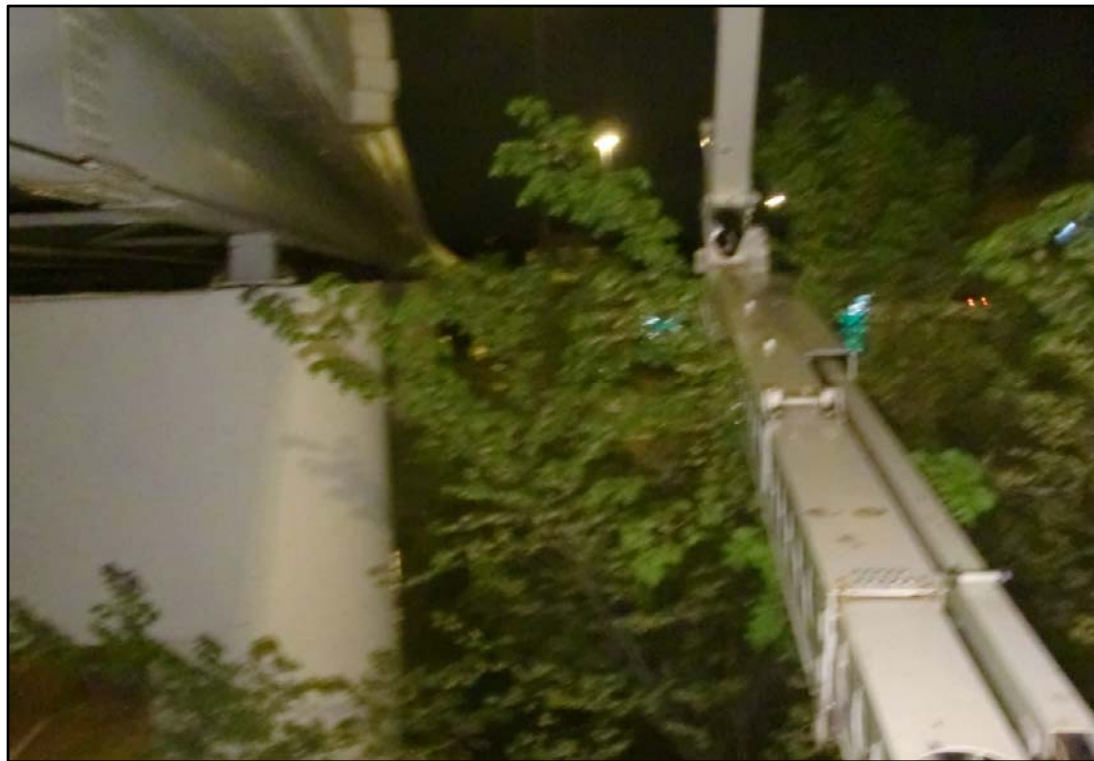
Photo 41 – Tree Growth within I-71 Median Obstructing Snoopers Access.
