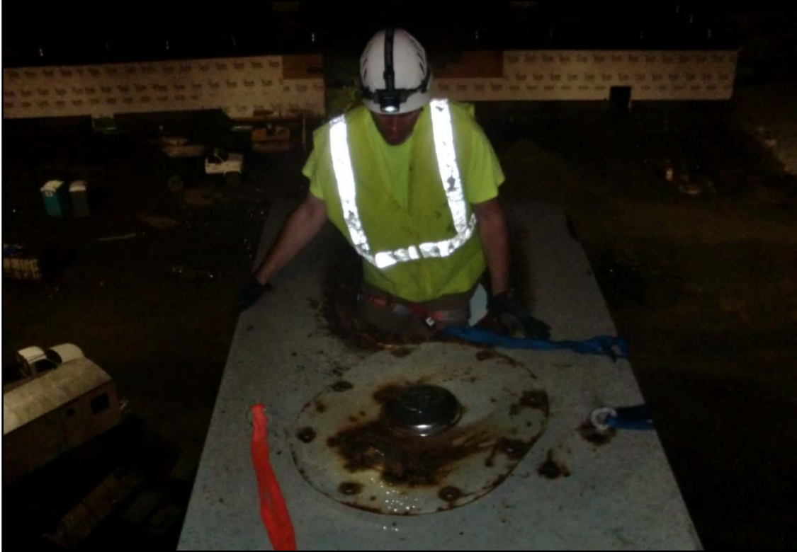
Photo 4 – Climbing Procedure to Pier 17 Steel Box Interior.
