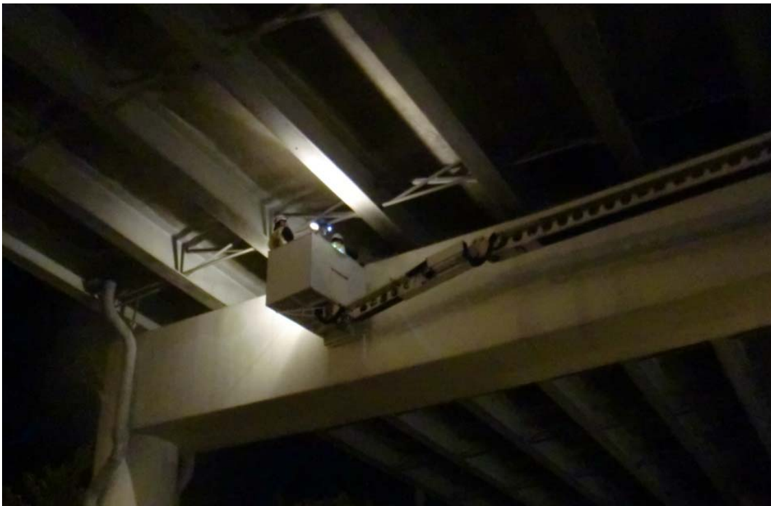
Photo 3 – Snooper Access Using Bucket Mounted Lamps.
