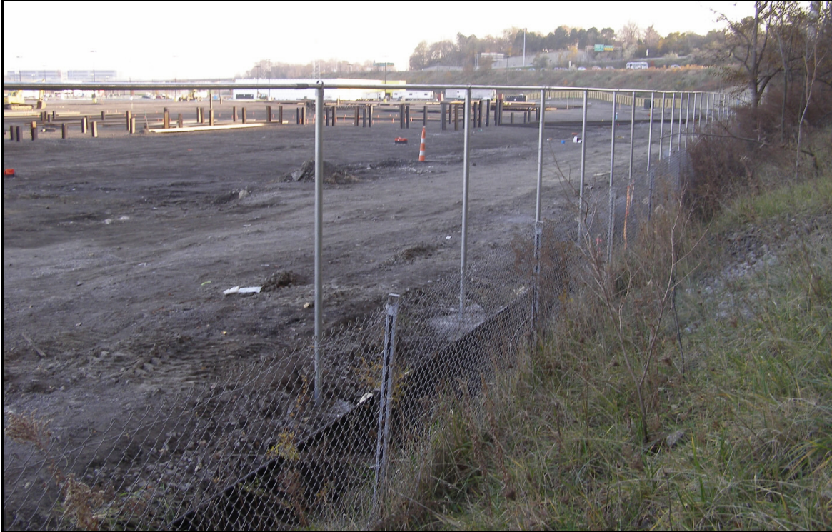
Photo 48 – New 8-Ft. High Chain Link Fence for Steelyard Commons
