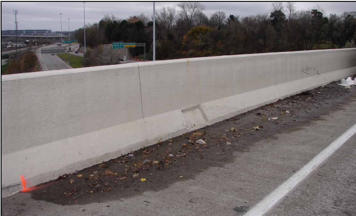
Photo 14 – Standing Water in Right Gutterline, Span 3
