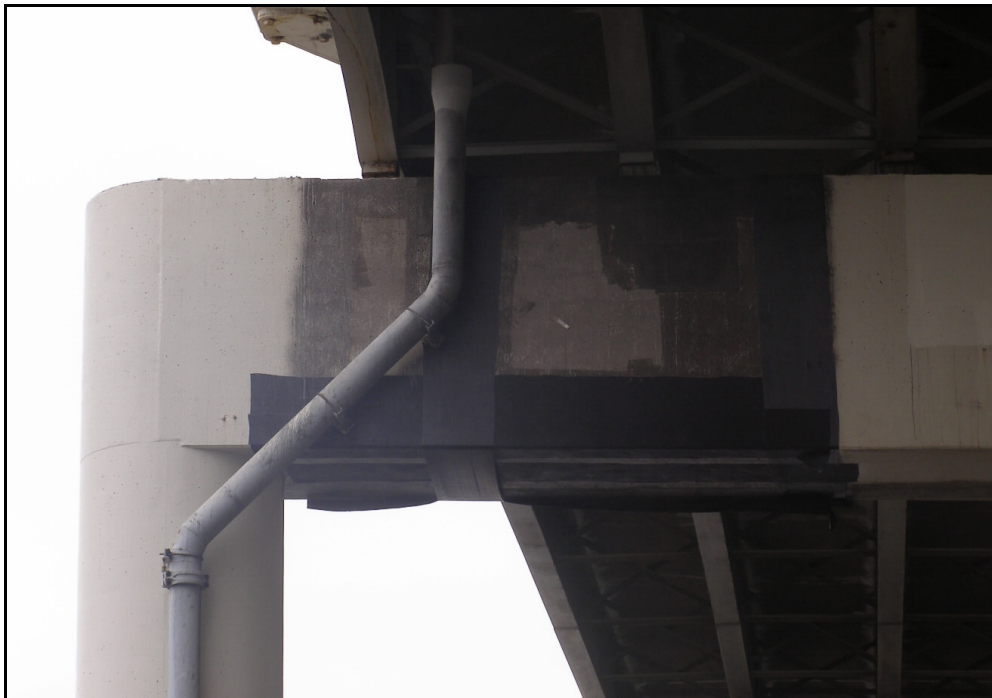
Photo 35 – Installation of External Carbon Fiber Reinforcement, Pier 11
