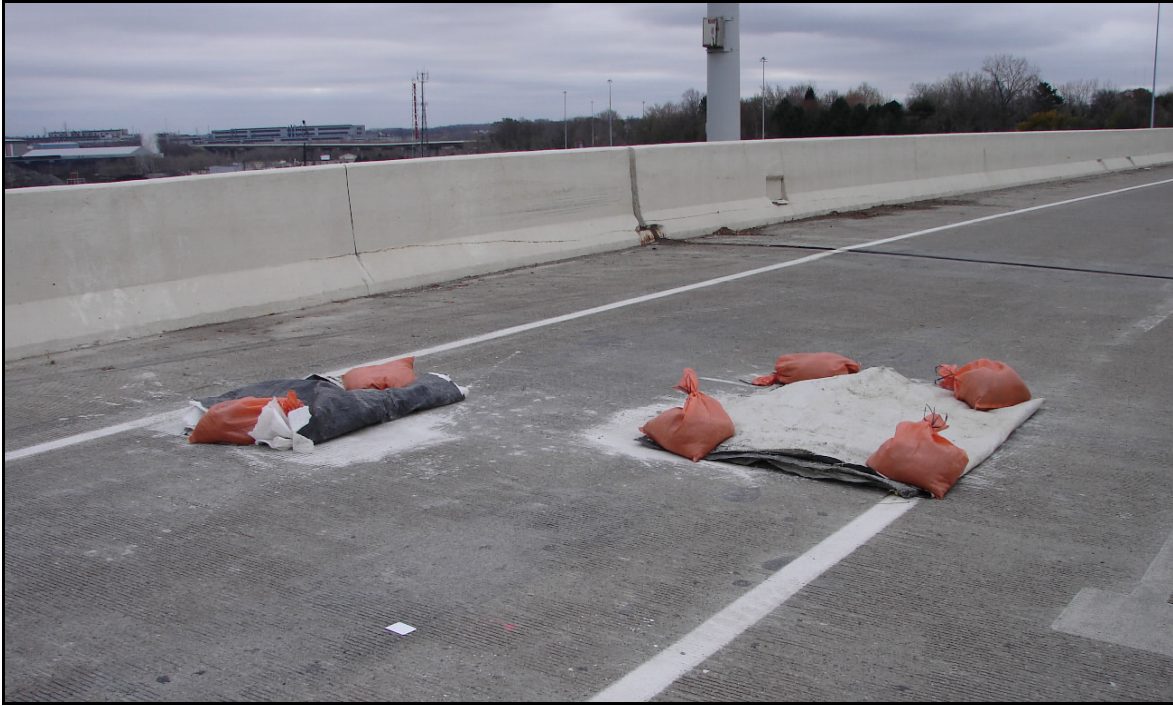
Photo 4 – Wearing Surface Repair, Lane 4, Span 7
