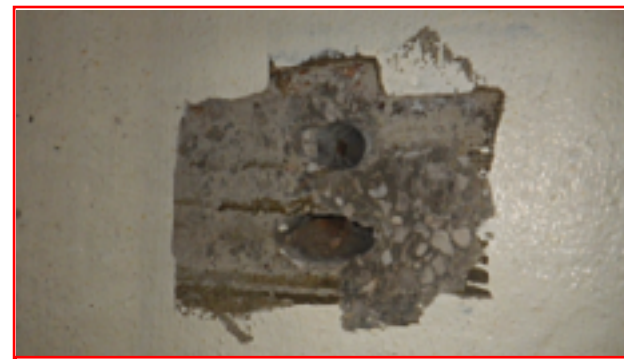
Two holes drilled through barrier.
