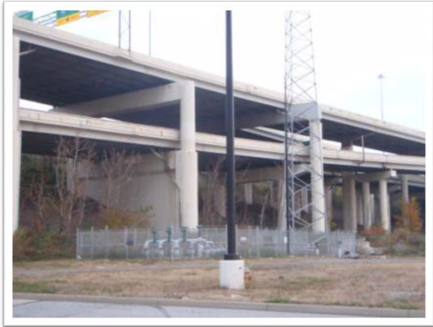
Elevation View Looking West
