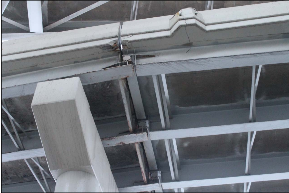
Photo 8 – Edge of Floor Slabs at Expansion Joint 2BW.
