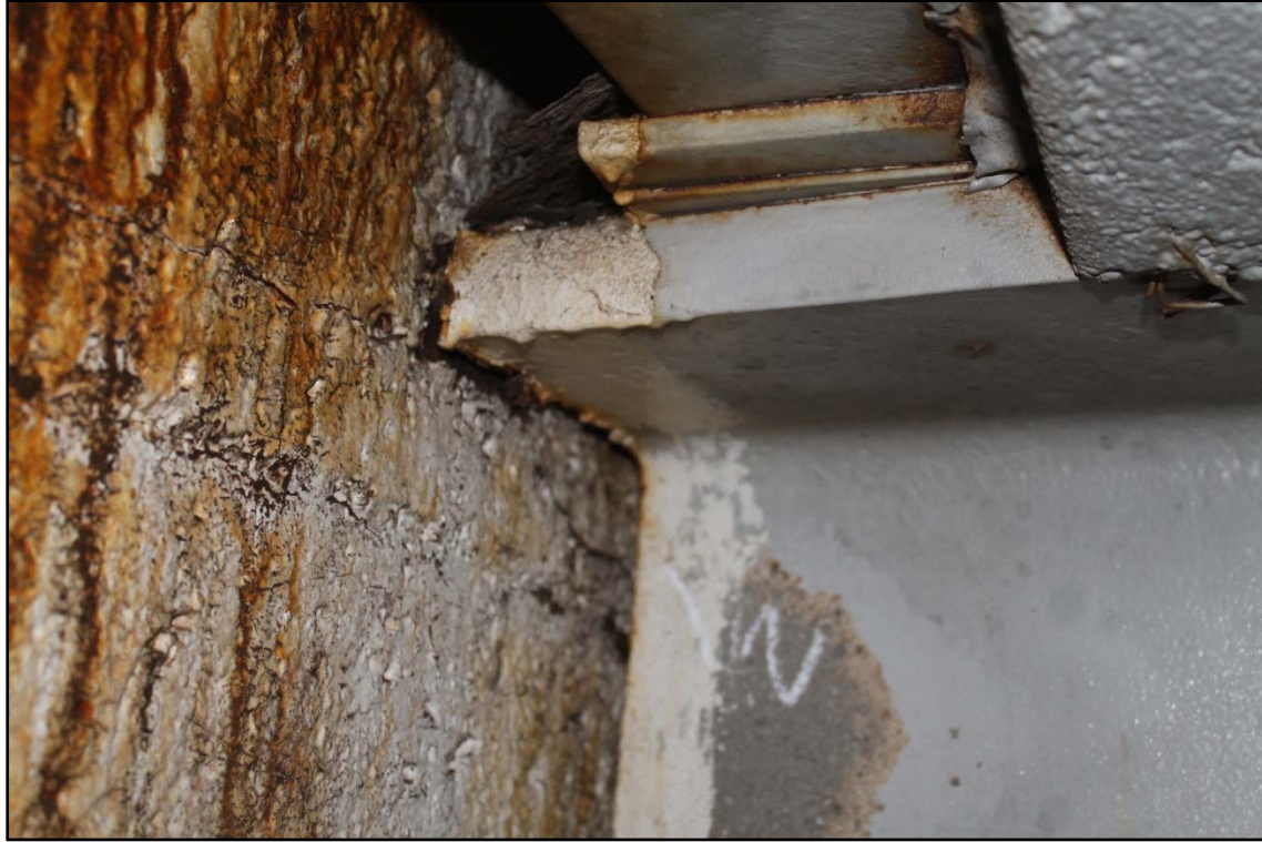
Photo 26 – Backwall Contact with Beam C, Abutment BW.
