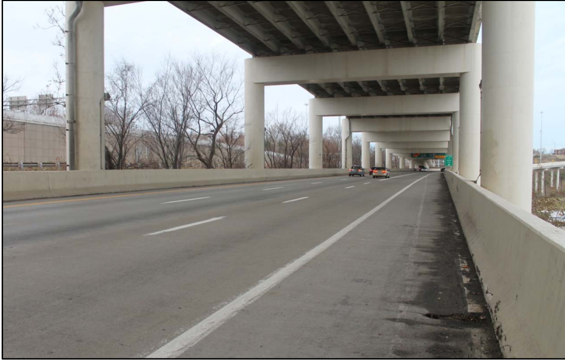
Photo 2– SR 176 Bridge Deck View.
