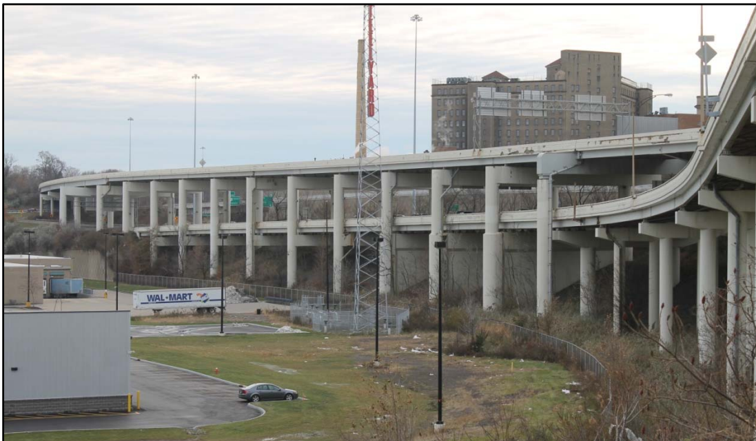
Photo 1– SR 176 Bridge East Elevation.
