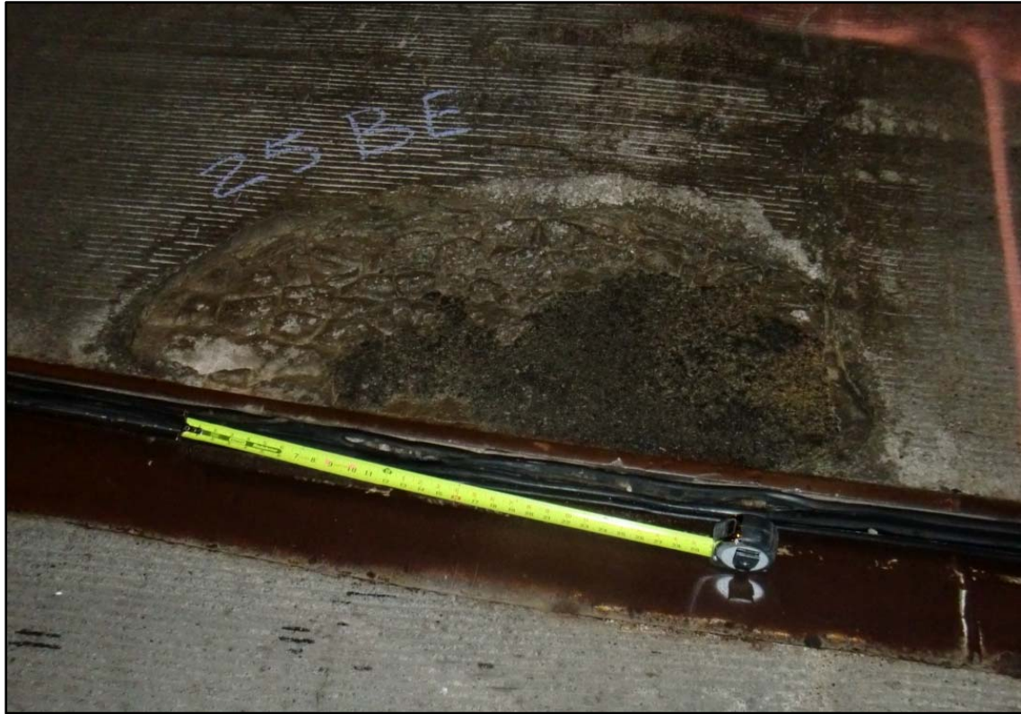
Photo 10 – Wearing Surface Patch, Span 25BE.
