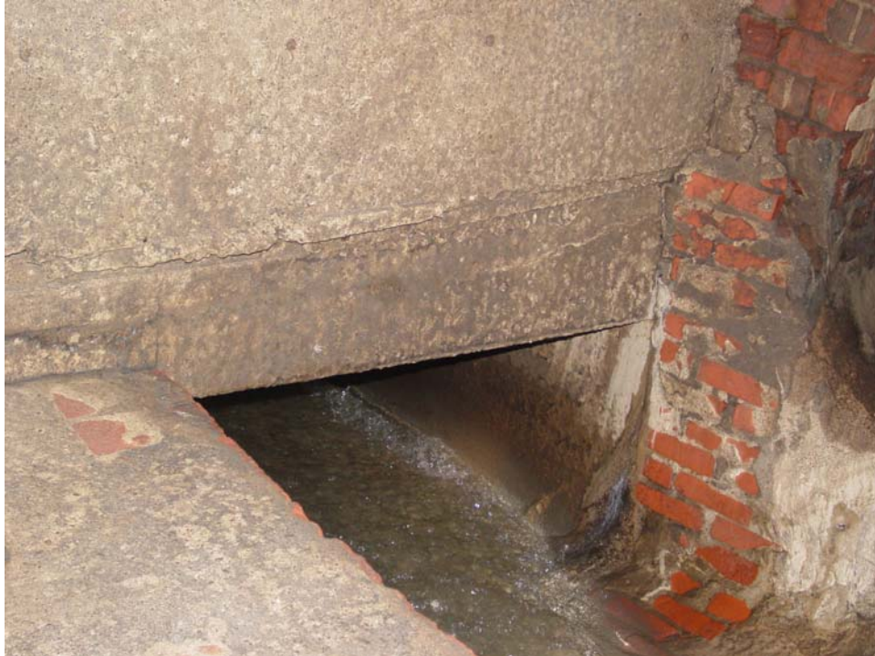
Photo 3 – Facing northeast. View of the diversion channel at weir wall, water exiting beneath Finish (north) wall.
