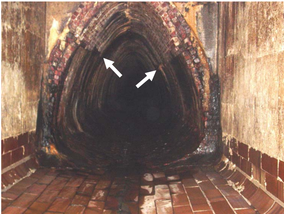
Photo 12 – Facing East. View of abutting brick and concrete culvert sections. Note line of water infiltration along horizontal cracks.
