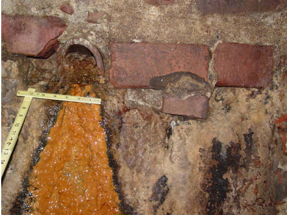
Photo 9 – Facing North. View of intersecting 4” diameter clay pipe drain. Note missing brick and concrete patching.
