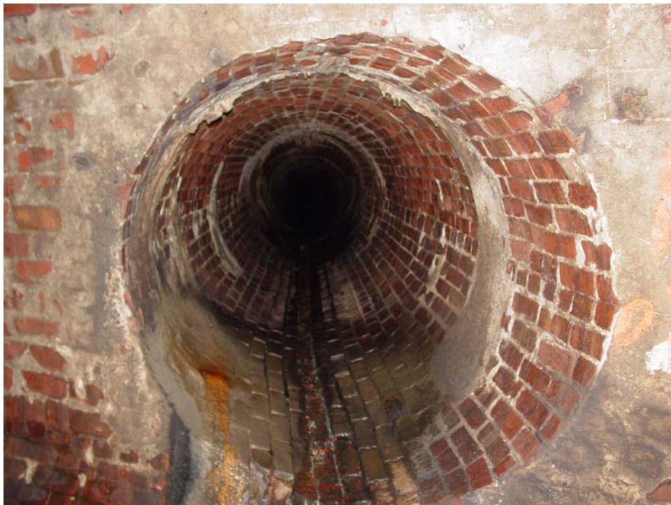
Photo 8 – Facing South. View of intersecting 48” diameter brick sewer.
