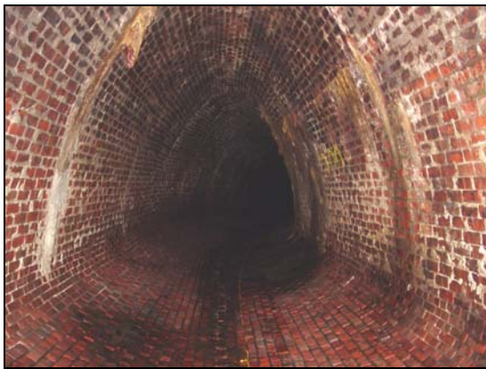
General View of Culvert
