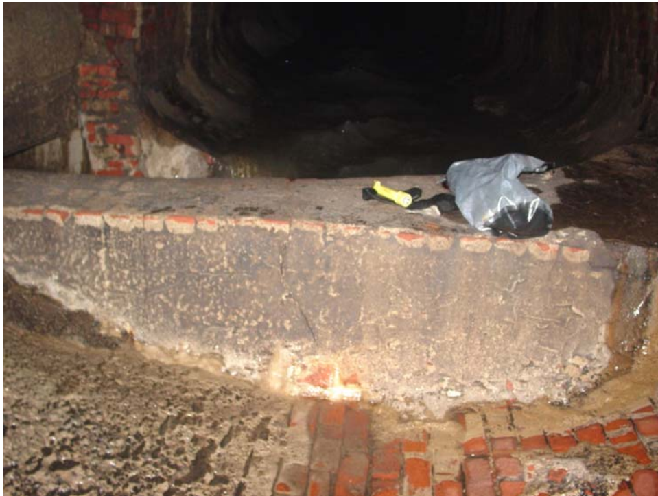
Photo 2 – Facing East. Elevation view of the weir wall near 49 th Street manhole.
