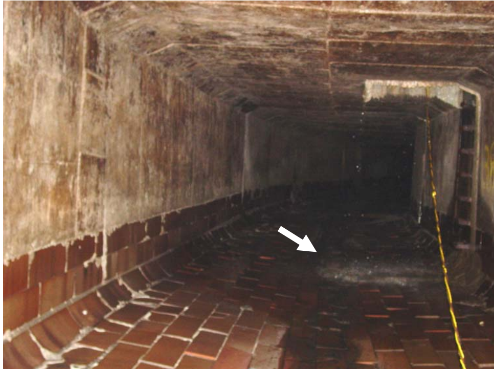
Photo 13 – Facing East. View of concrete and tile culvert section and the Mittal Steel manhole entrance ladder. Note heavy water intrusion.
