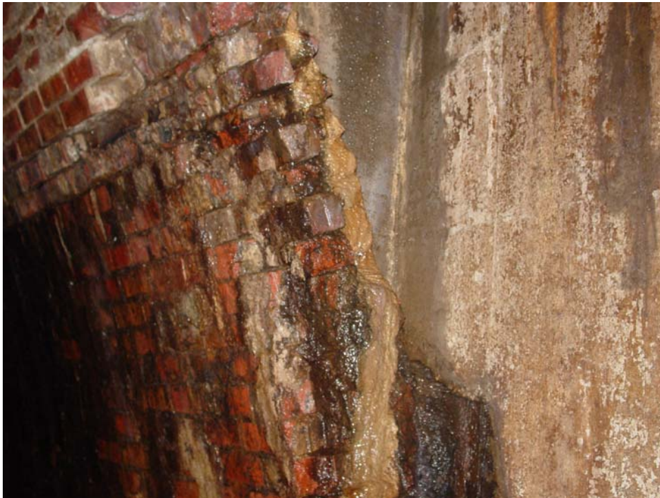
Photo 10 – Facing Southeast. View of abutting brick and concrete culvert sections along Start (South) wall.
