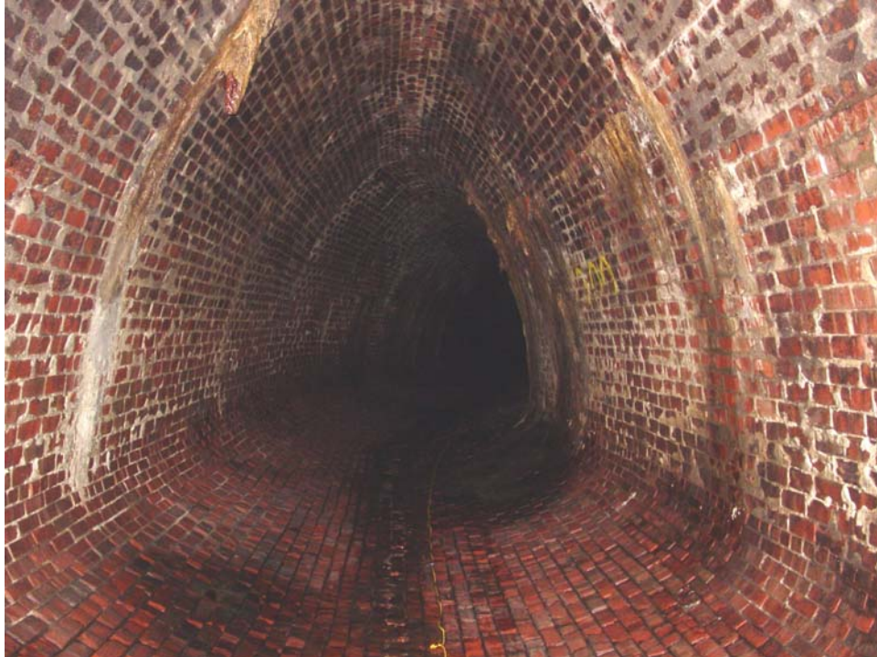
Photo 7 – Facing West. Note water infiltration and heavy efflorescence along each wall.
