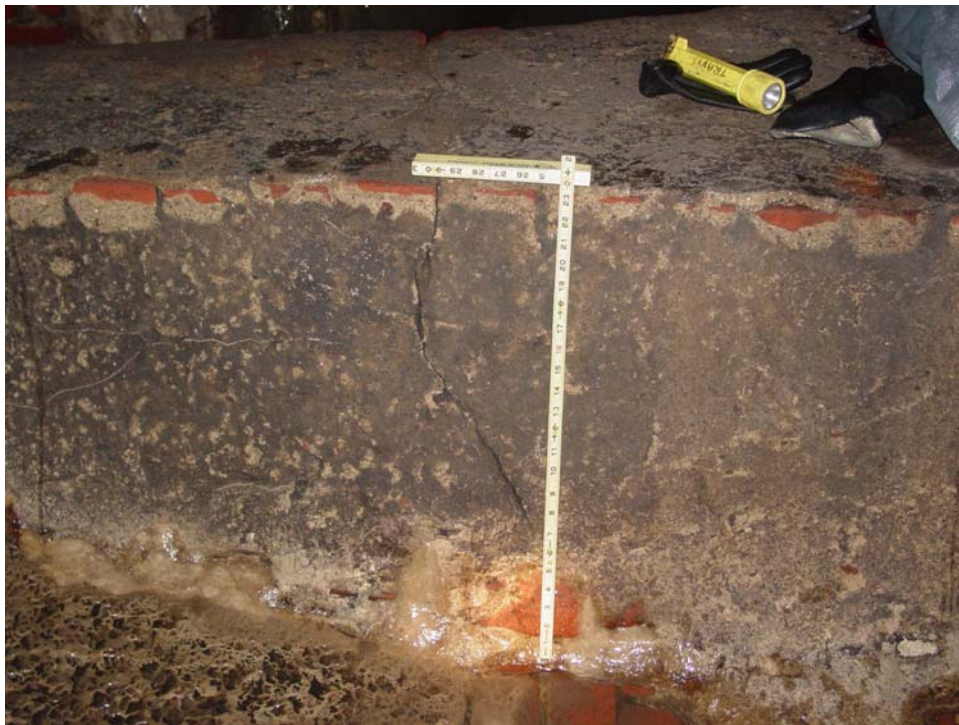
Photo 4 – Facing East. View of crack through weir wall.
