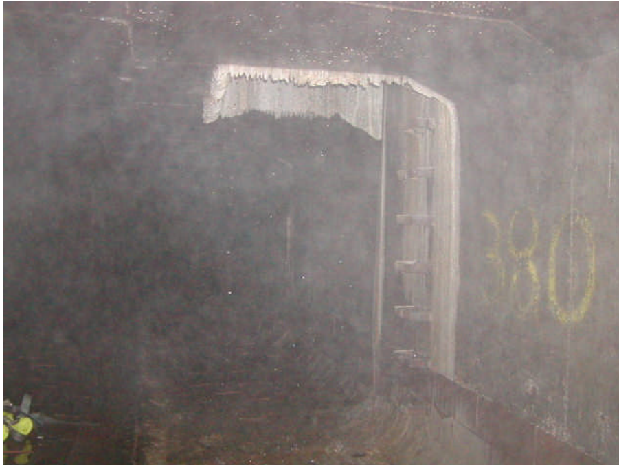
Photo 3. Mittal Street manhole entrance ladder.
