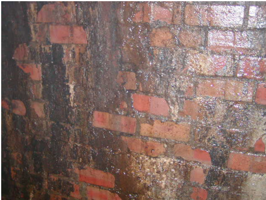
Photo 4. Typical brick culvert wall.
