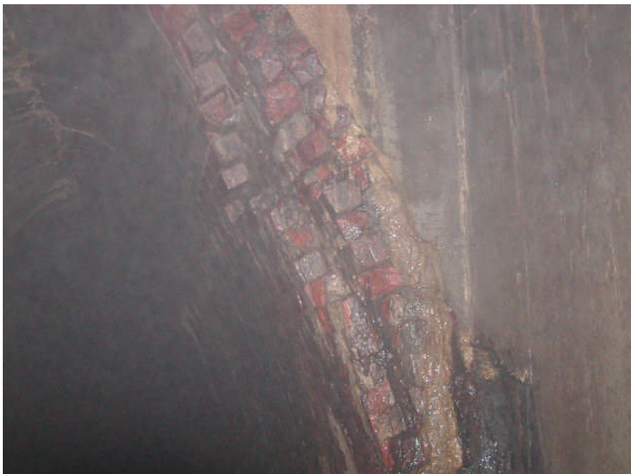
Photo 12. Joint between brick and concrete portion of the culvert.
