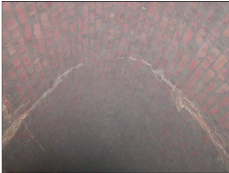
General Elevation View
