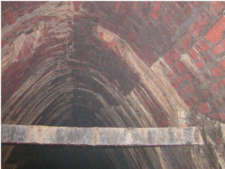
Photo 10. Brick roof and horizontal beam.
