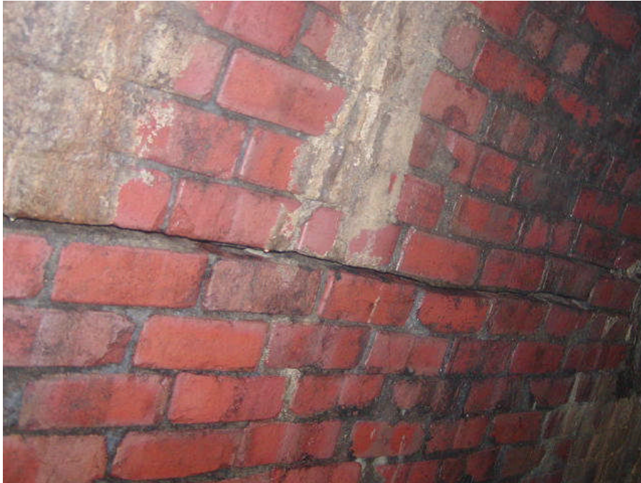
Photo 11. Missing mortar between bricks.
