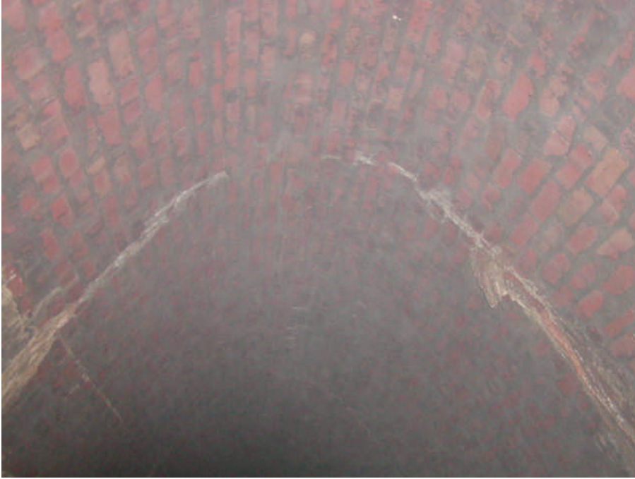
Photo 5. Culvert brick roof.
