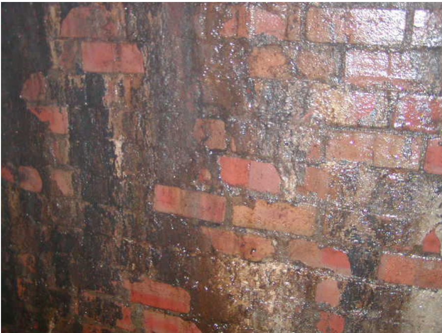
Photo 4. Typical brick culvert wall.
