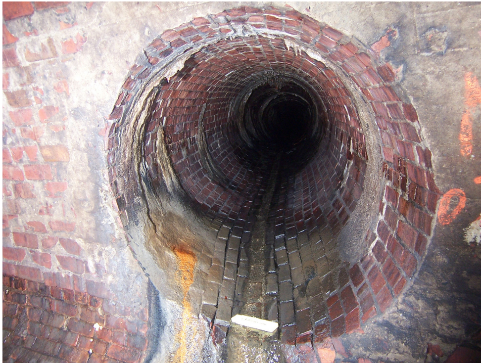
Photo 9 – Facing South at 160 feet from the Arcelor Mittal Steel entry point. 48-inch diameter brick incoming pipe.
