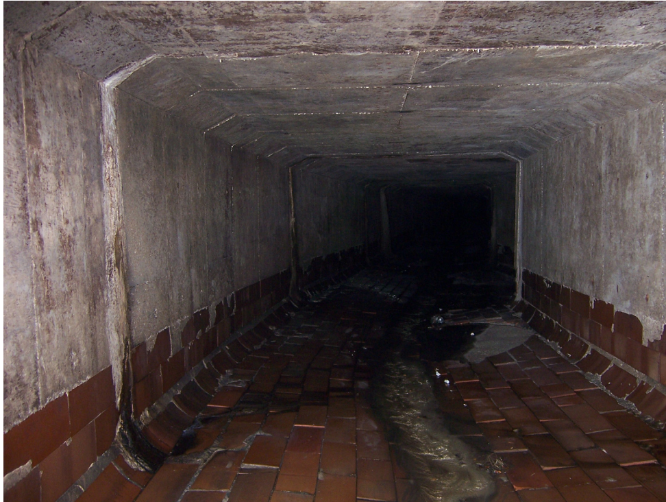
Photo 15 – Facing West. Concrete and Tile Culvert.
