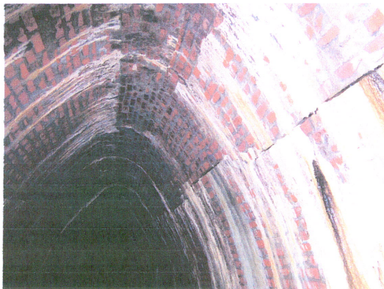
General View of Brick Culvert
