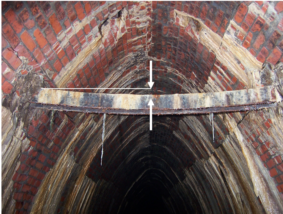
Photo 5 – Facing West at 370 feet from the Arcelor Mittal Steel entry point. Steel Beam with approximate 2-inch deflection.
