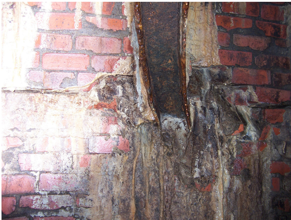
Photo 6 – Facing North. Area where the Steel Beam penetrates the brick wall.
