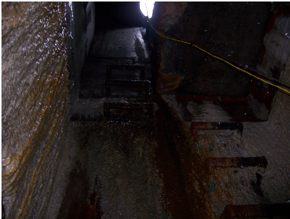
Photo 16 – Facing up at entry point. Note the offset in the ladder rungs.
