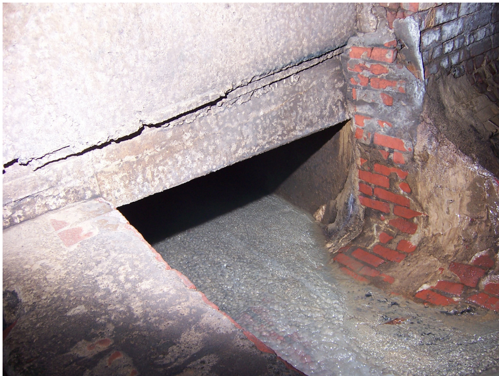
Photo 4 – Facing Northeast. Diversion Channel at the Weir Wall with water exiting beneath North Wall.
