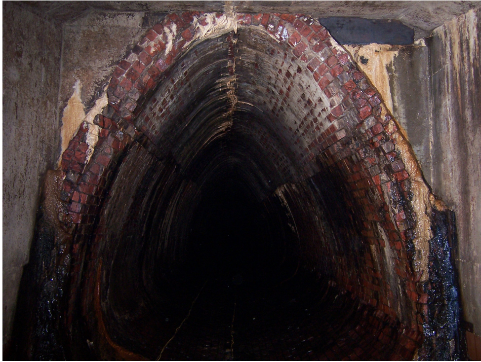
Photo 13 – Facing East. Transition from Concrete to Brick Culvert.
