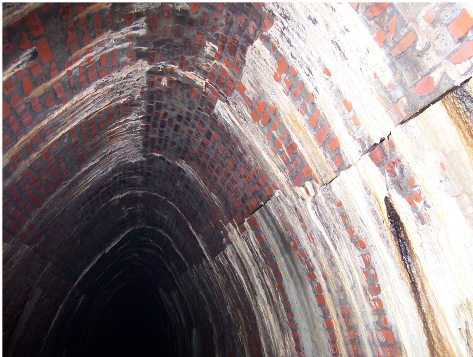
Photo 8 – Facing West at 365 feet from the Arcelor Mittal Steel entry point. Horizontal Mortar Joint Cracks with infiltration and efflorescence.
