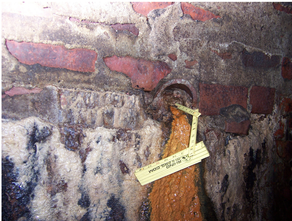
Photo 9 – Facing South at 160 feet from the Arcelor Mittal Steel entry point. 48-inch diameter brick incoming pipe.
