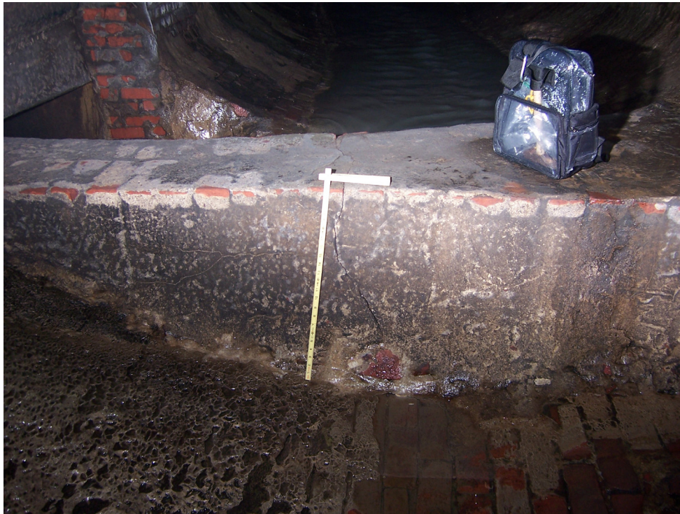
Photo 3 – Facing East. Weir Wall with 1/16-inch through crack.
