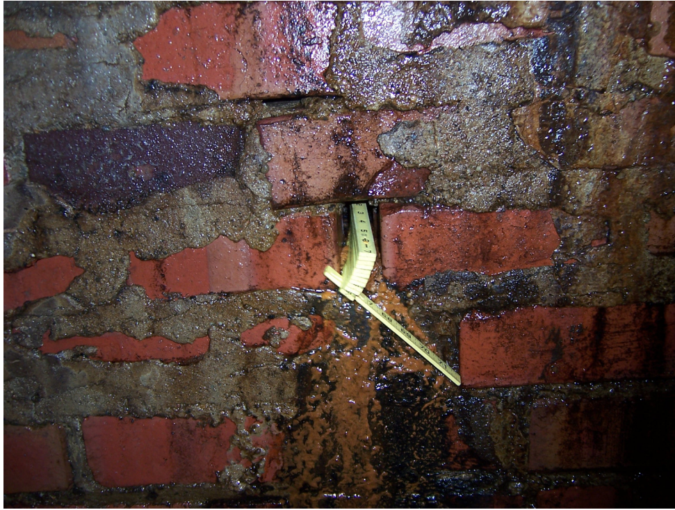
Photo 11 – Facing North at 150 feet from the Arcelor Mittal Steel entry point. 2-inch wide x 3-inch high hole in first layer of brick.
