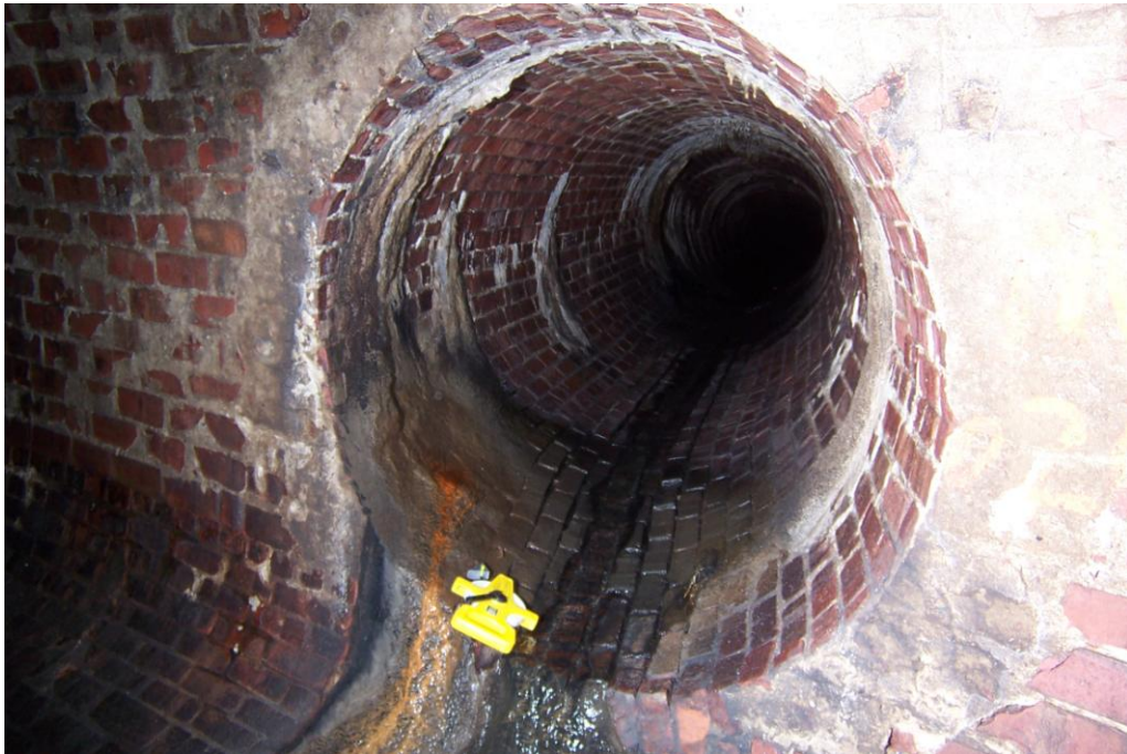
Photo 9 – Facing South 290 feet from the entry manhole. 48-inch diameter brick incoming pipe.
