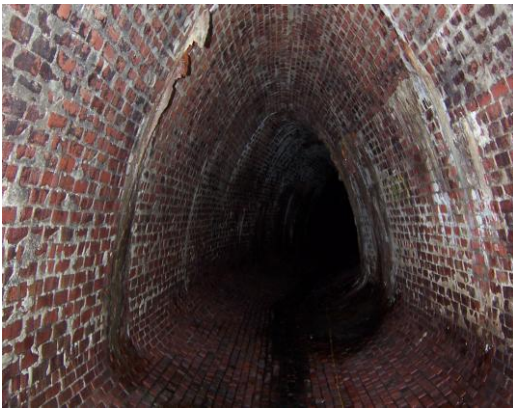
General View of Brick Culvert
