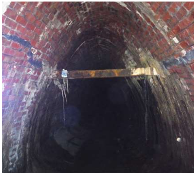
(General View of Brick Arch Structure)
