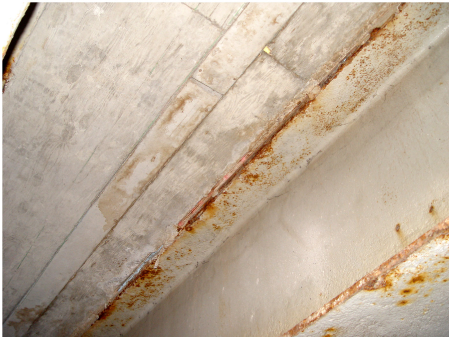
1808311 11_7_05 P3 plywood cast into floor.jpg
