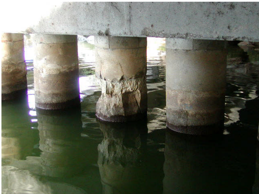
Photo 4. Typical Section Loss.
