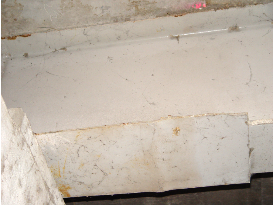
1808311 10_5_05 P6 bent beam 5 cover plate.jpg
