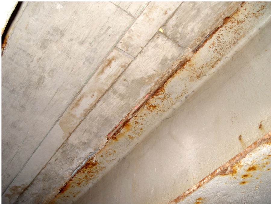
1808311 11_7_05 P3 plywood cast into floor.jpg
