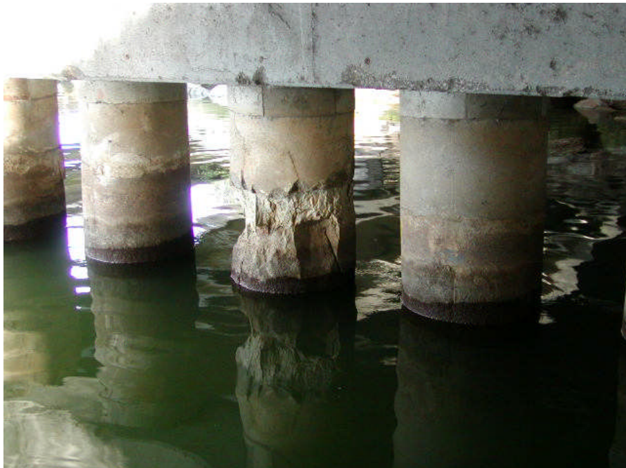
Photo 4. Typical Section Loss.
