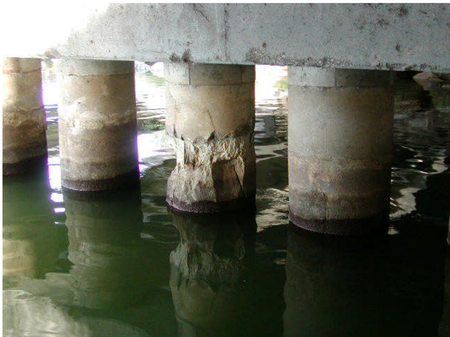
Photo 4. Typical Section Loss.
