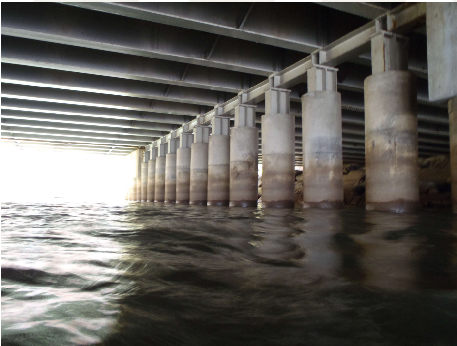
Photo 2 - Typical Bent Configuration, Bent 1
