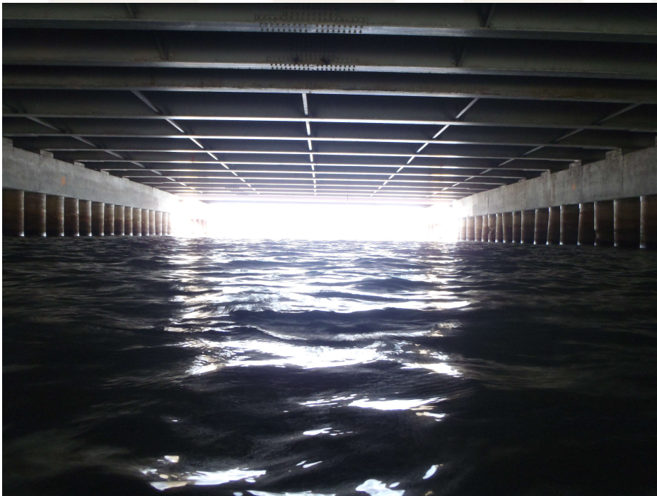
Photo 4 - Channel View Looking Downstream (North)
