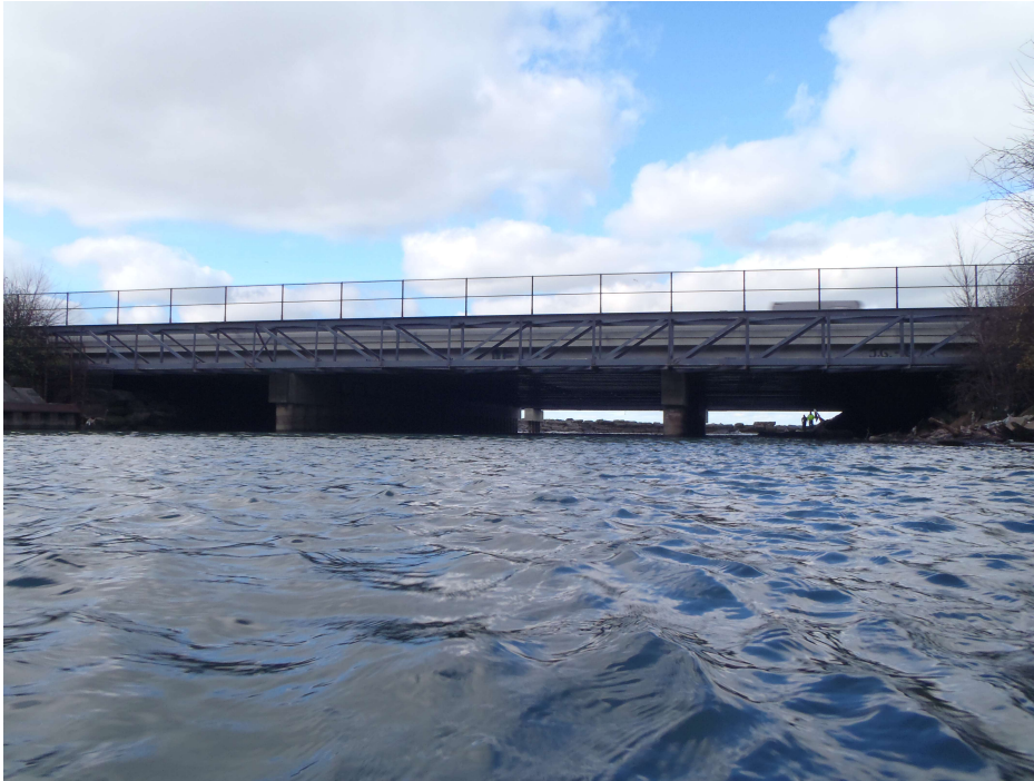
Photo 1 - Upstream (South) Fascia Looking North
