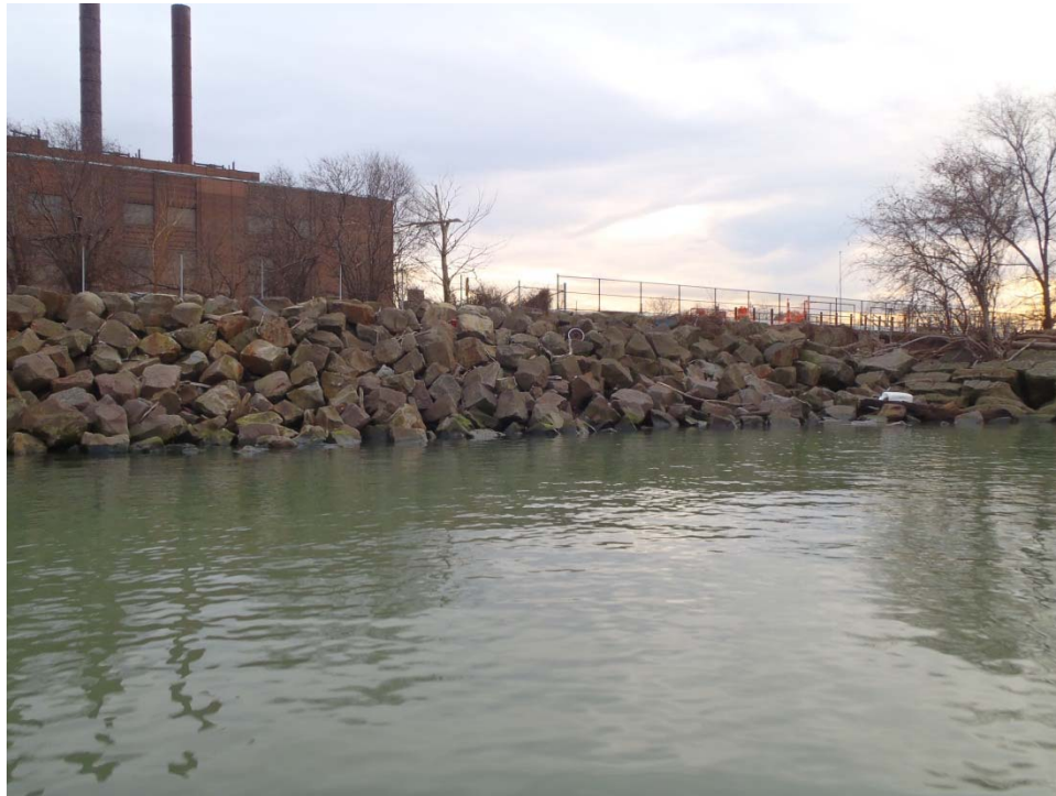
Photograph 2: Riprap revetment east of the intake canal, typical of all riprap revetments.
