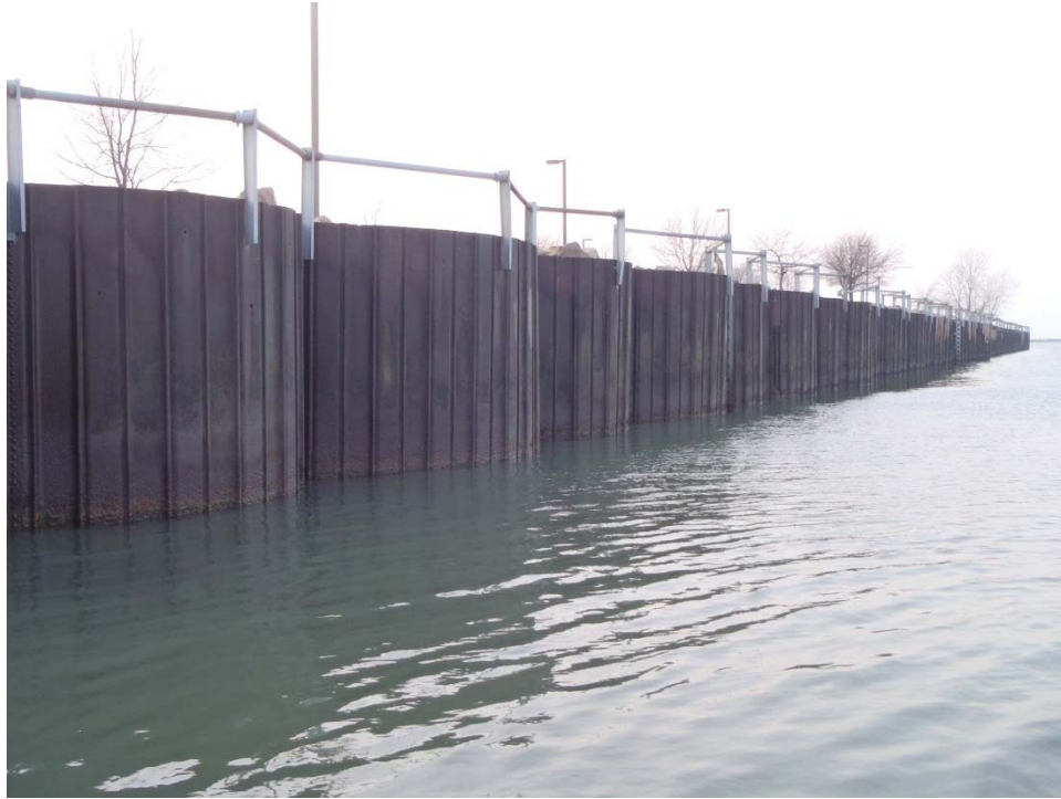
Photograph 1: West Bulkhead looking northwest, typical of the West and South Bulkheads.
