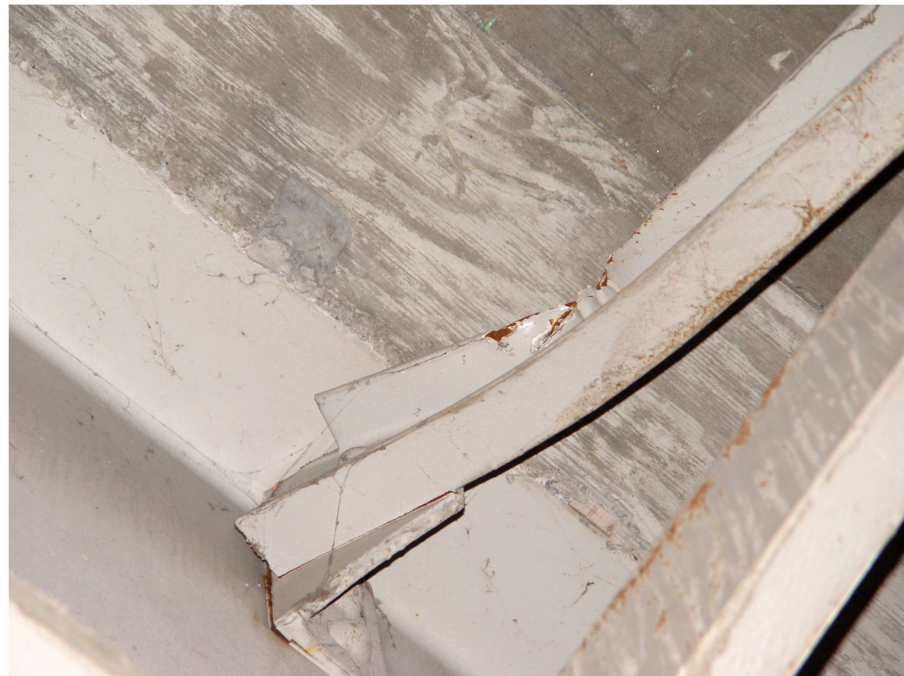
1808745 10_5_05 P4 bent crossframe channel.jpg
