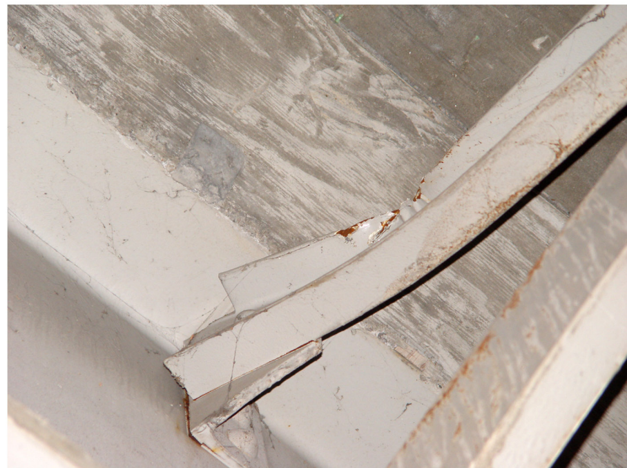
1808745 10_5_05 P4 bent crossframe channel.jpg
