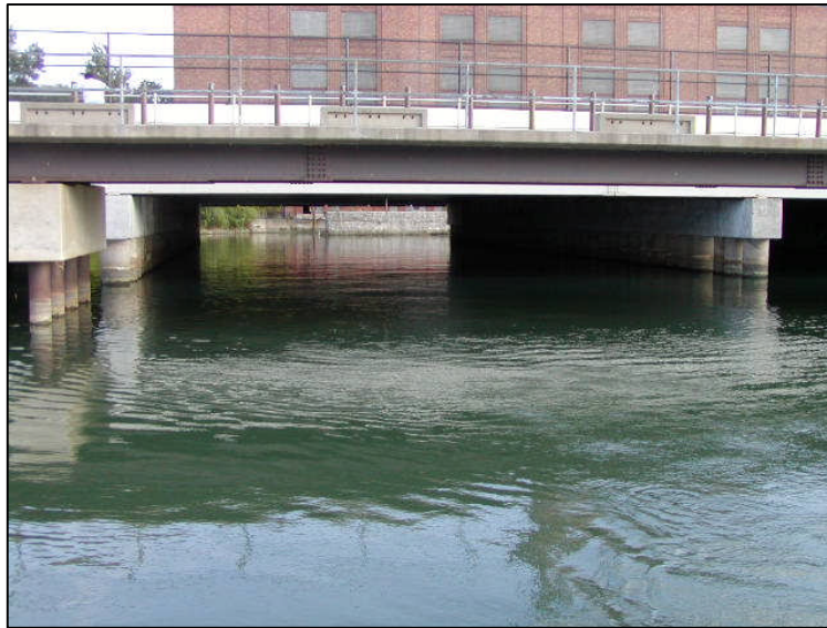
General Elevation View
