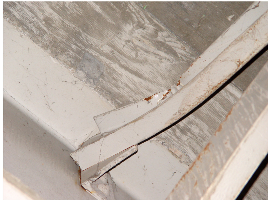
1808745 10_5_05 P4 bent crossframe channel.jpg
