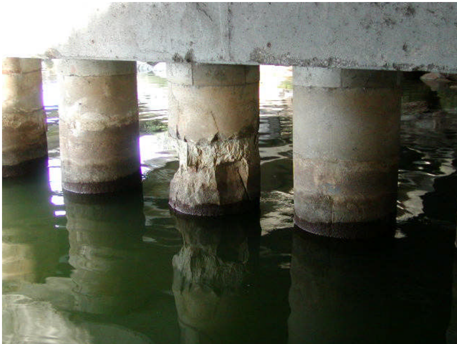
Photo 4. Typical Section Loss.
